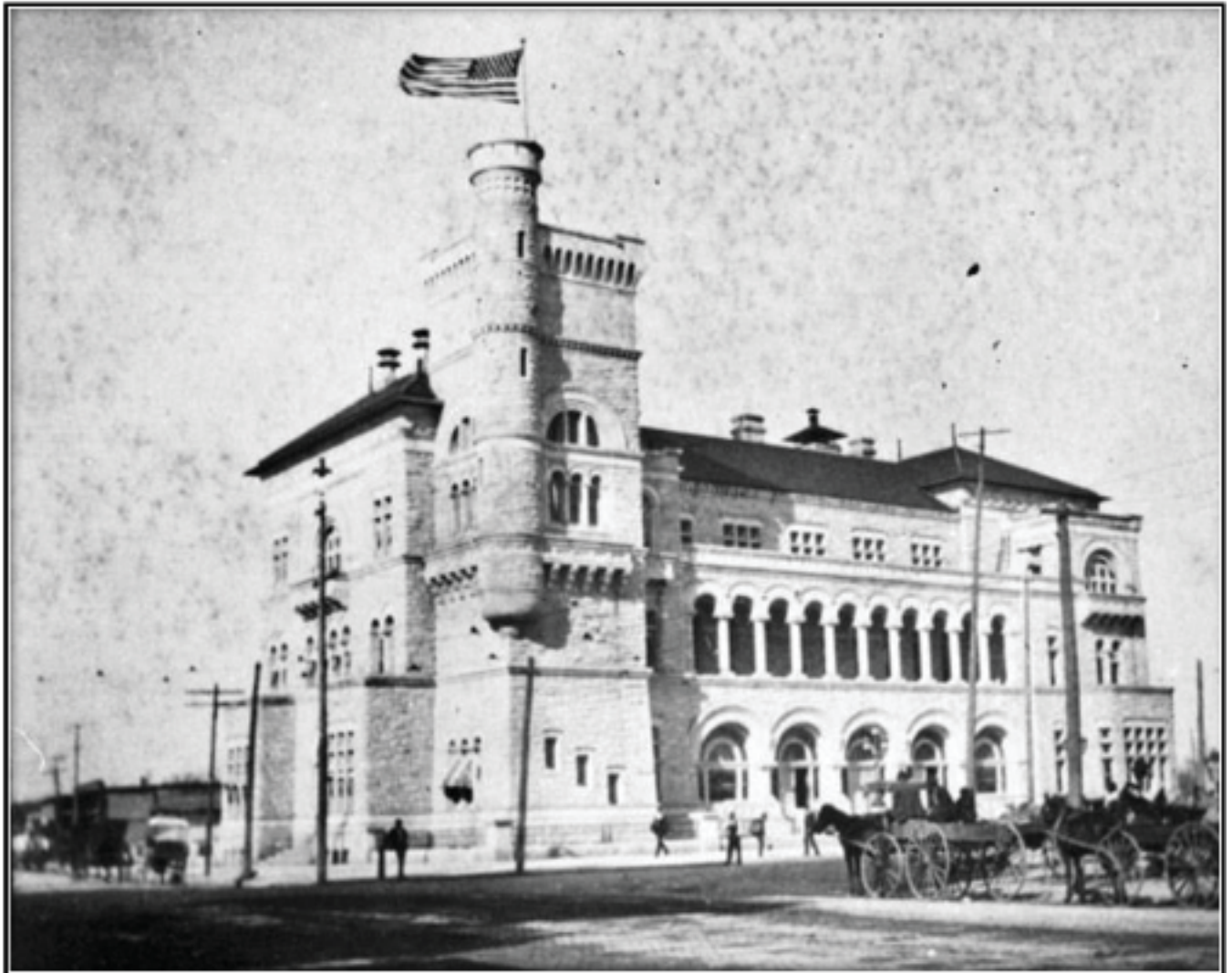
Figure 6-4. West and south elevations of the Federal Building and Post Office on Alamo Plaza, San Antonio, Texas, ca. 1893, courtesy of the San Antonio Conservation Society, University of Texas at San Antonio, Special Collections Department, Digital Collections, General Photograph Collection Image Number 076-0525.
