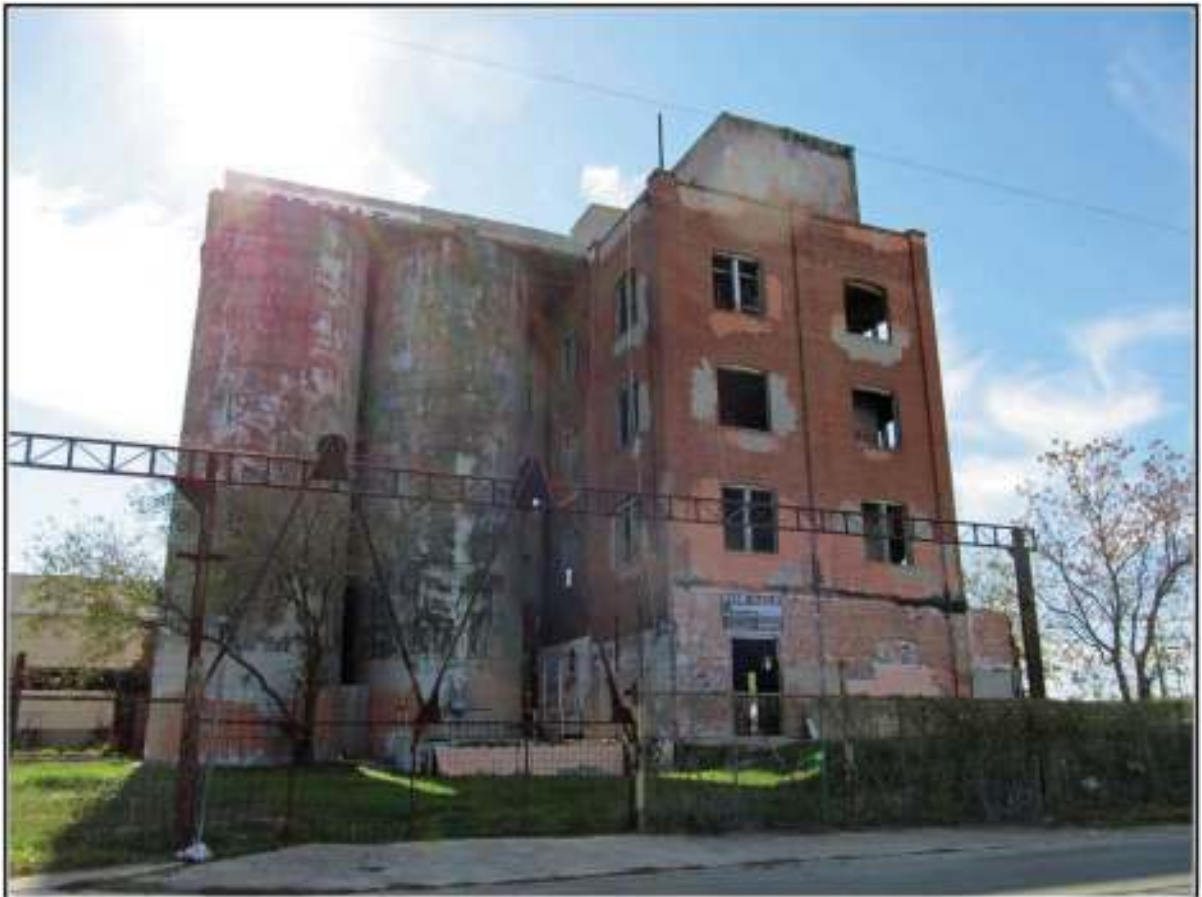
Figure H-20. The Tamalina Milling building in 2011 at the corner of Colima and Medina.
