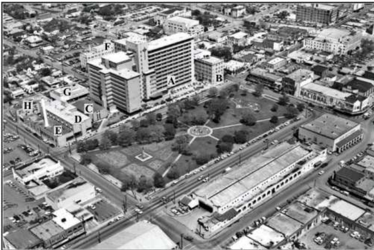
Figure 3-25. Aerial view of Santa Rosa Medical Center, Milam Park, and Municipal Market, San Antonio, Texas, March 1968: A. 1960 Hospital, B. 1921 East Wing, C. 1953 Chapel, D. 1961 Convent, E. 1948 Boiler House, F. 1937 School of Nursing, G. 1961 Radiology Building, H. 1949 Laundry Building. (Ray Howell Photograph Collection, MS 354, UTSA Libraries Special Collections, Image Identifier H-5124-089).
