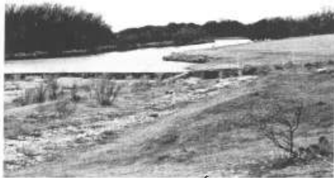
Figure 63. White's Dam across Spring Creek was originally constructed of wood in 1885. After this concrete dam was built around 1906, the opening on the right diverted water into the Twin Mountain Ditch.
