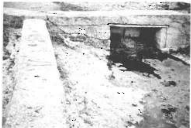
Figure 64. This 5-foot opening in White's Dam provided the headwaters for the Twin Mountain Ditch. (Note the impressions in the concrete.)
