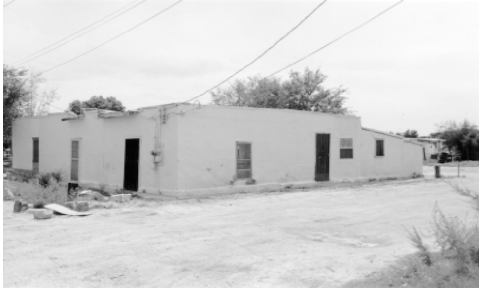
Figure 7. Additions on the building at 1519 Camino Barrial.
