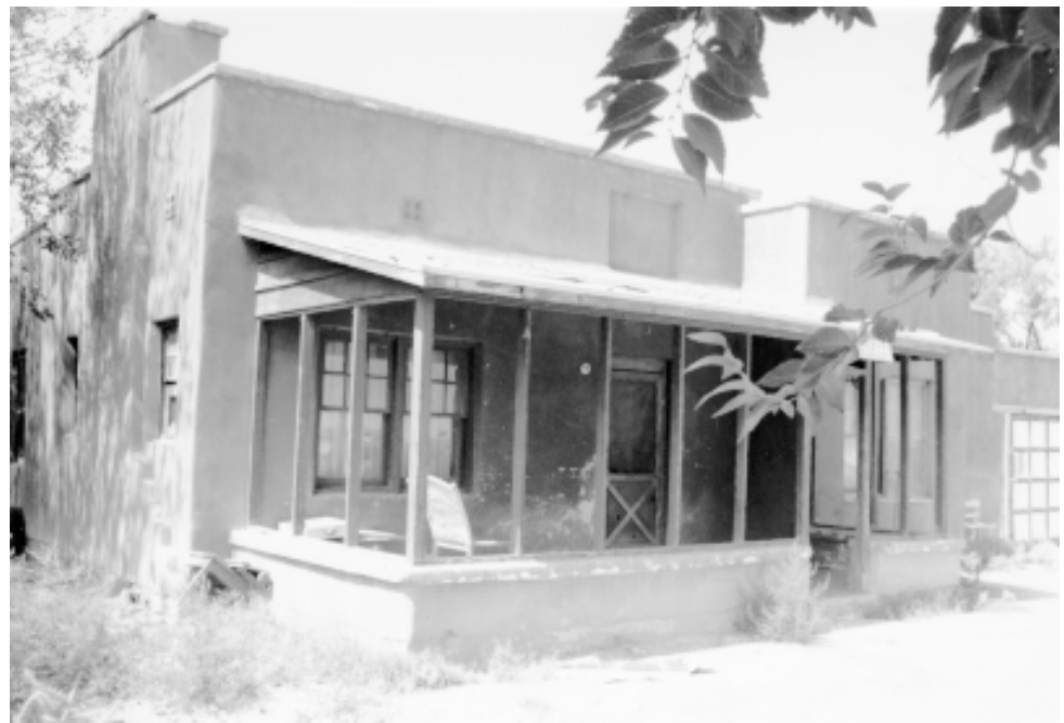
Figure 24. 12300 Camino de la Rosa Road.
