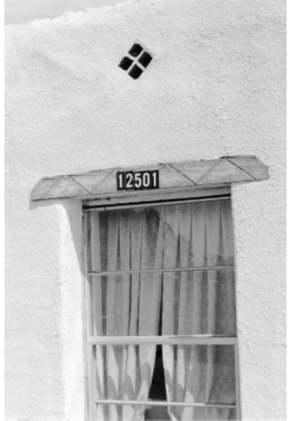
Figure 9. Wood lintels with geometric patterns at 12501 Caballero Road.
