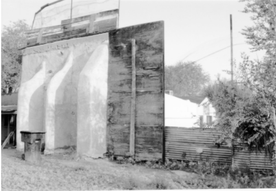
Figure 37. Buttresses supporting a wall of the ballcourt.
