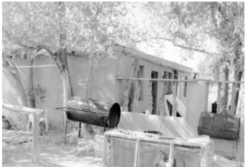
Figure 13. 12296 Cinnabar Road, southern building.
