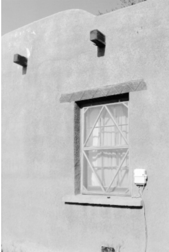
Figure 8. Wood lintels with geometric patterns at 12337 Socorro Road.
