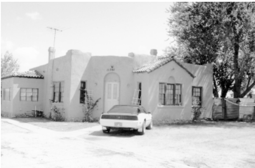
Figure 11. Decorative clay tile roof at 11391 North Loop Road.
