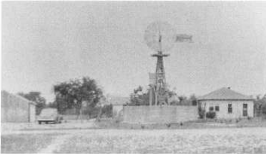
Figure 18. Zacatosa Ranch headquarters, about 1942. Looking west. (Laughlin AFB Base Properties Files).
