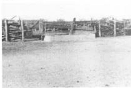
Figure 24. The system of corrals built of horizontal boards and stacked logs (Laughlin AFB Base Properties Files).
