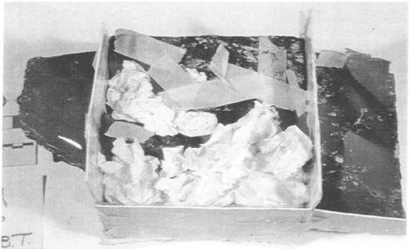
FIGURE 13. Top view of the void area in the muntin filled with acid-free tissue paper prior to infilling with RTV738.
