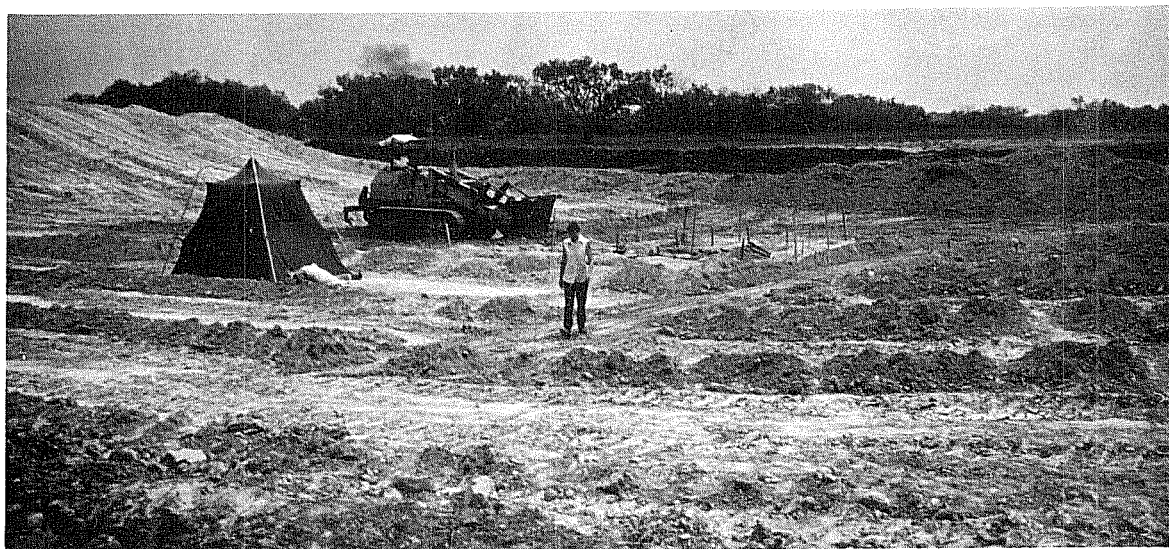
Figure 4. La Paloma Site . Heavy equipment used to remove overburden and define limits of mammoth at site 1. Note the shallow occurrence of the bone array.
