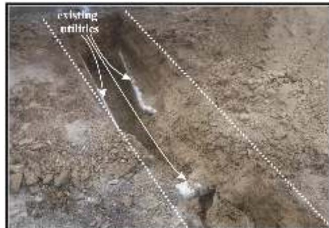
Figure 4-5. Gas line trench, view southwest.
