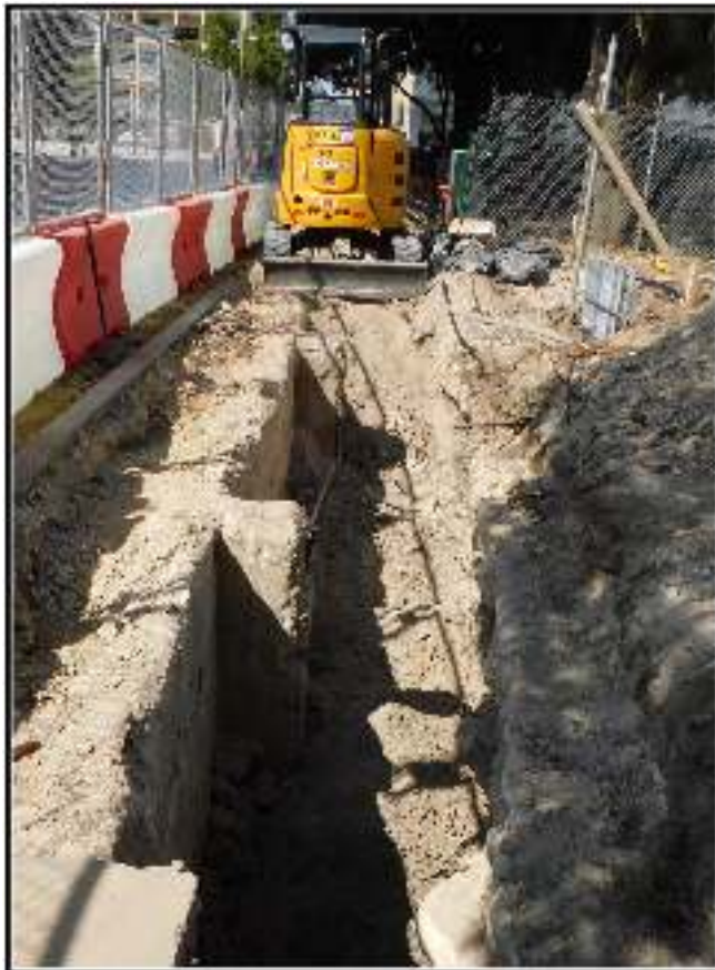
Figure 4-1. Electrical line project area along the east side of N. Flores Street. Note concrete pier and beam footings for the Majestic Theatre, site 41BX2347 (view north).
