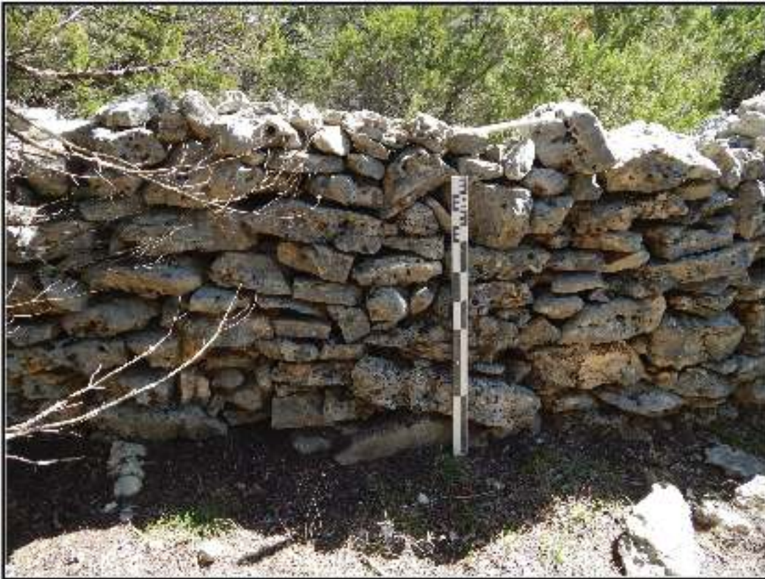
Figure 4-45. Intact portion of Rock Wall Section 1, 41BX1211.
