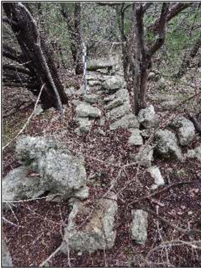
Figure 4-43. Partially intact segment of Rock Wall Section 1, 41BX1211. Note double-walled construction.
