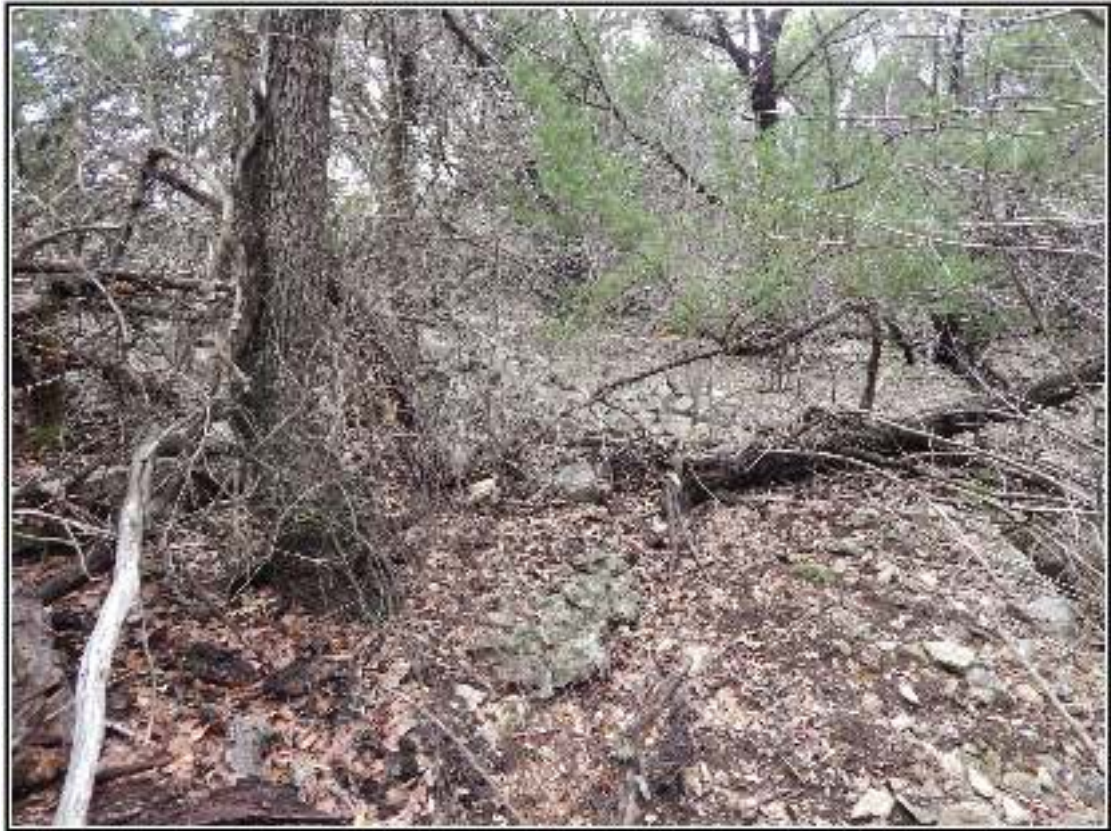
Figure 4-51. Rock Wall Section 5 damaged by drainage, 41BX1211.
