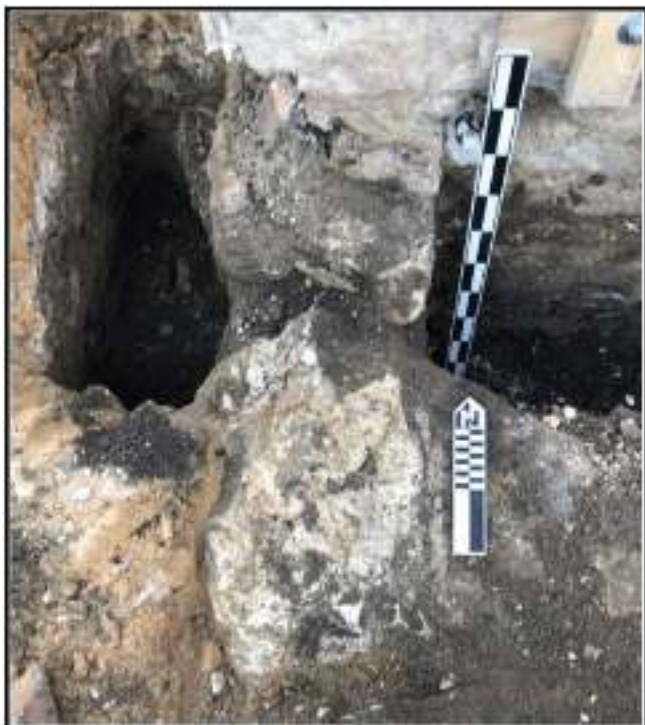
Figure 5-2. Feature 1, eastern wall foundation of original O'Hara House where it articulates with the remnant portion.
