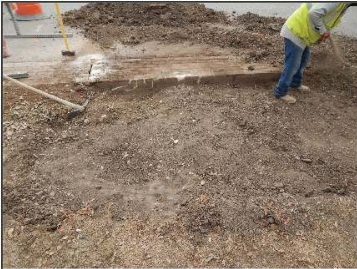
Figure 4-14. Graded area across from the entrance to Mission Espada.
