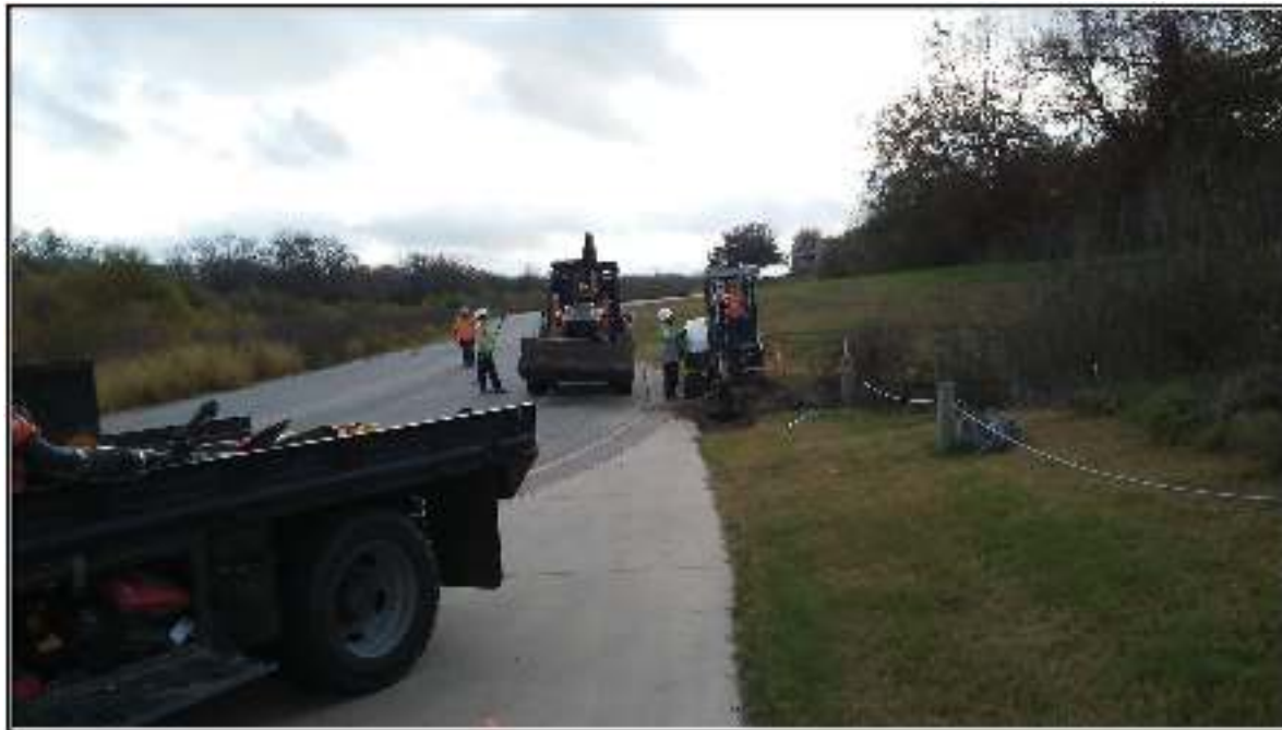
Figure 4-8. Beginning of excavations on Camino Coahuilteca (facing south).
