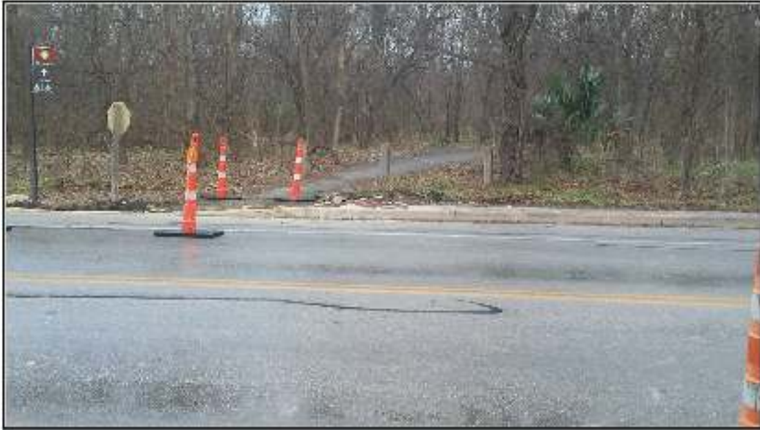
Figure 4-2. Excavation on west side of Padre Drive.
