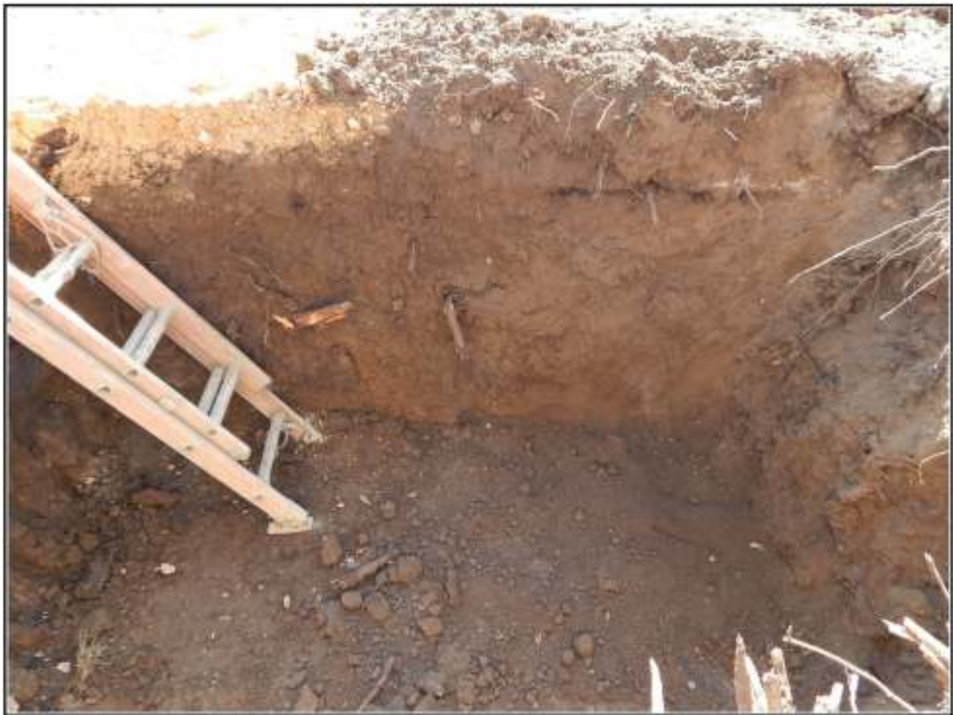
Figure 4-15. Trench excavation for pedestrian bridge crossing the Espada Acequia.
