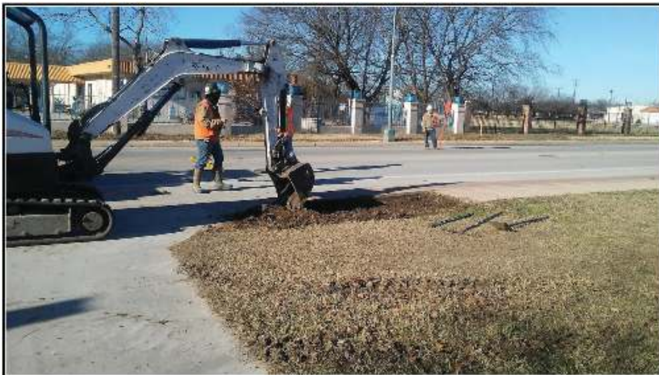
Figure 4-1. Beginning of excavations on Padre Drive (facing west).
