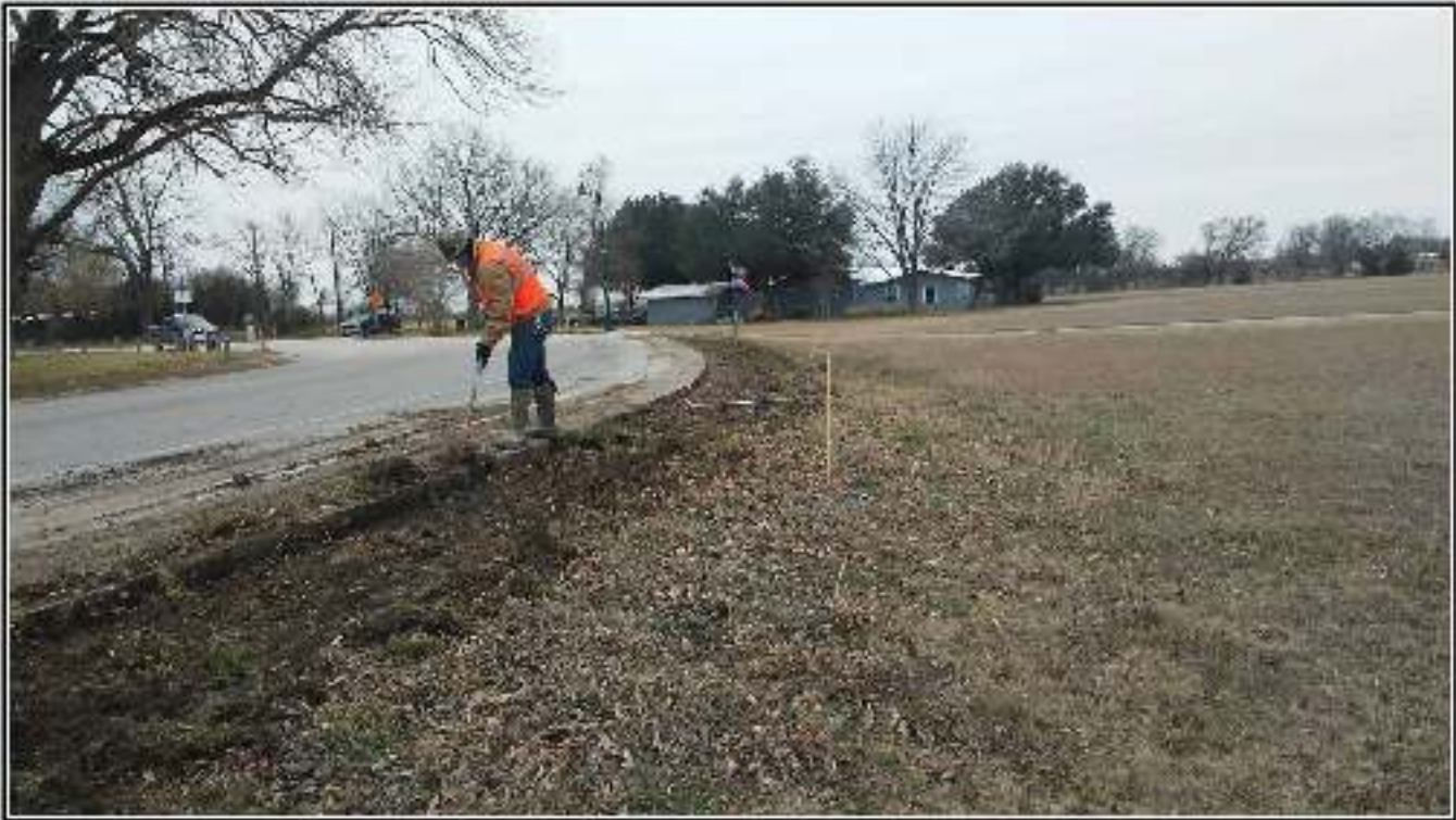
Figure 4-13. Excavations on the west side of Espada Road.
