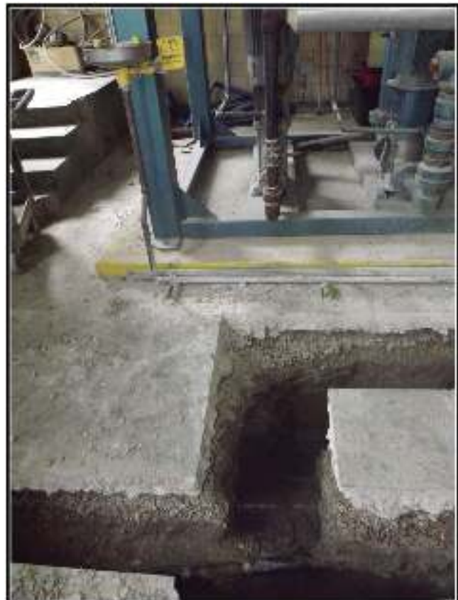
Figure 4-35. An example of trenching to repair pipes in the Boiler Room.
