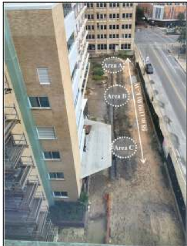
Figure 1-2. Aerial view of utility trench facing east, Areas A, B, and C noted.
