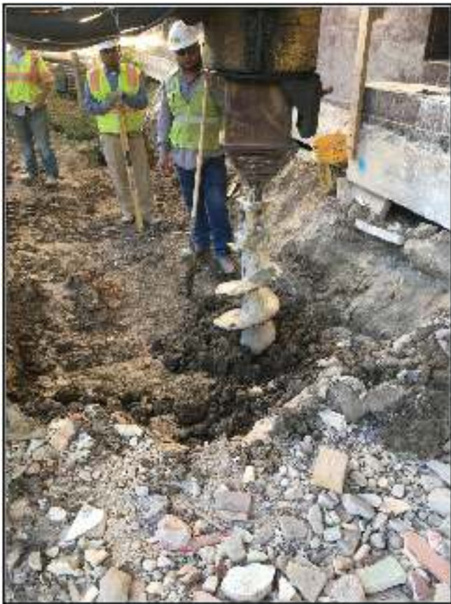
Figure 4-23. Core drilling on the location of Shovel Test 4.
