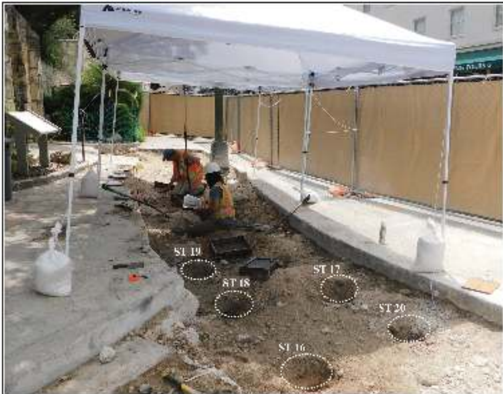
Figure 6-3. Excavation at east end of Area 1, ST 23 and ST 27 in progress.
