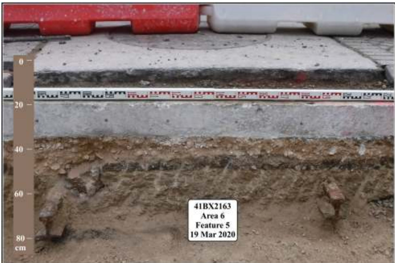
Figure 6-24. Feature 5, remnant of the Streetcar Rail System (41BX2163), view north.
