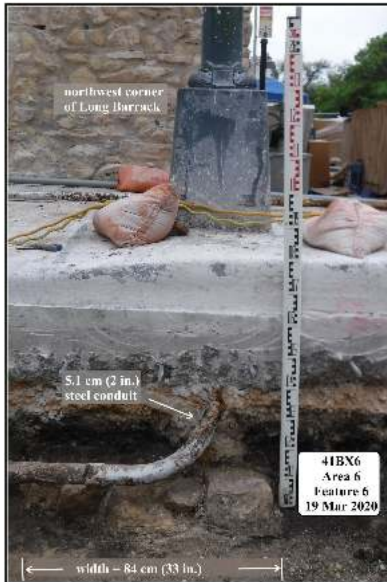
Figure 6-25. Feature 6, likely a Spanish Colonial wall footing (41BX6), view south.
