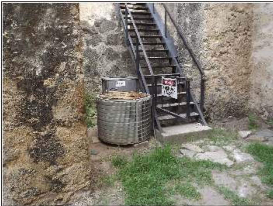
Figure 1-5. Former air conditioning and heating units in east portion of the APE.
