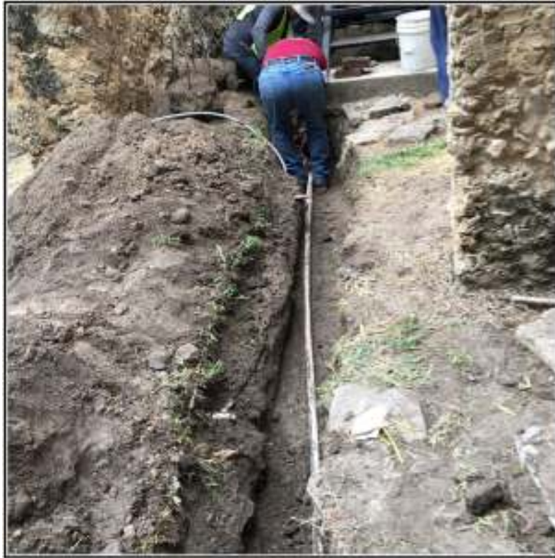
Figure 4-2. The excavated trench running to the east.
