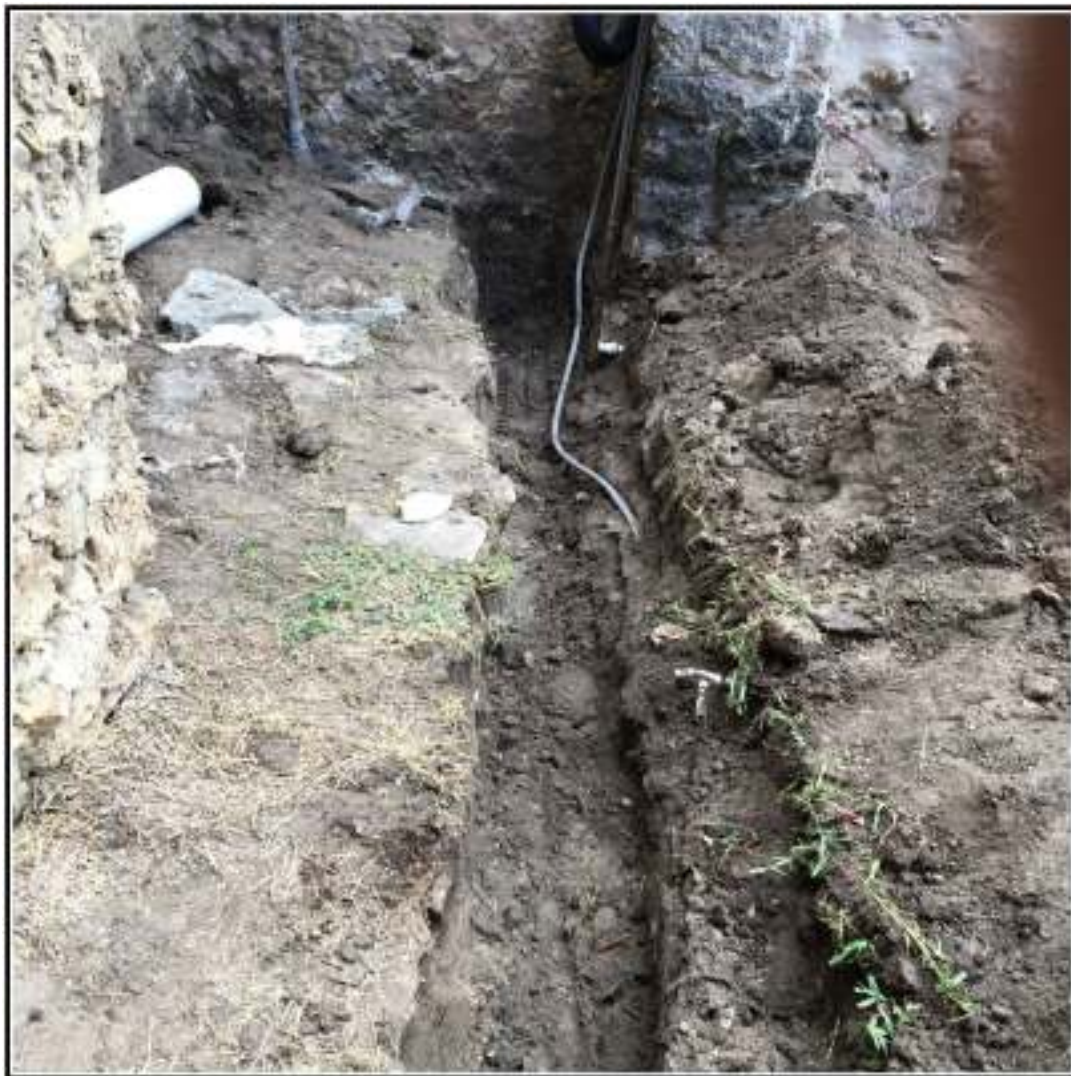
Figure 4-1. The excavated trench running to the west.
