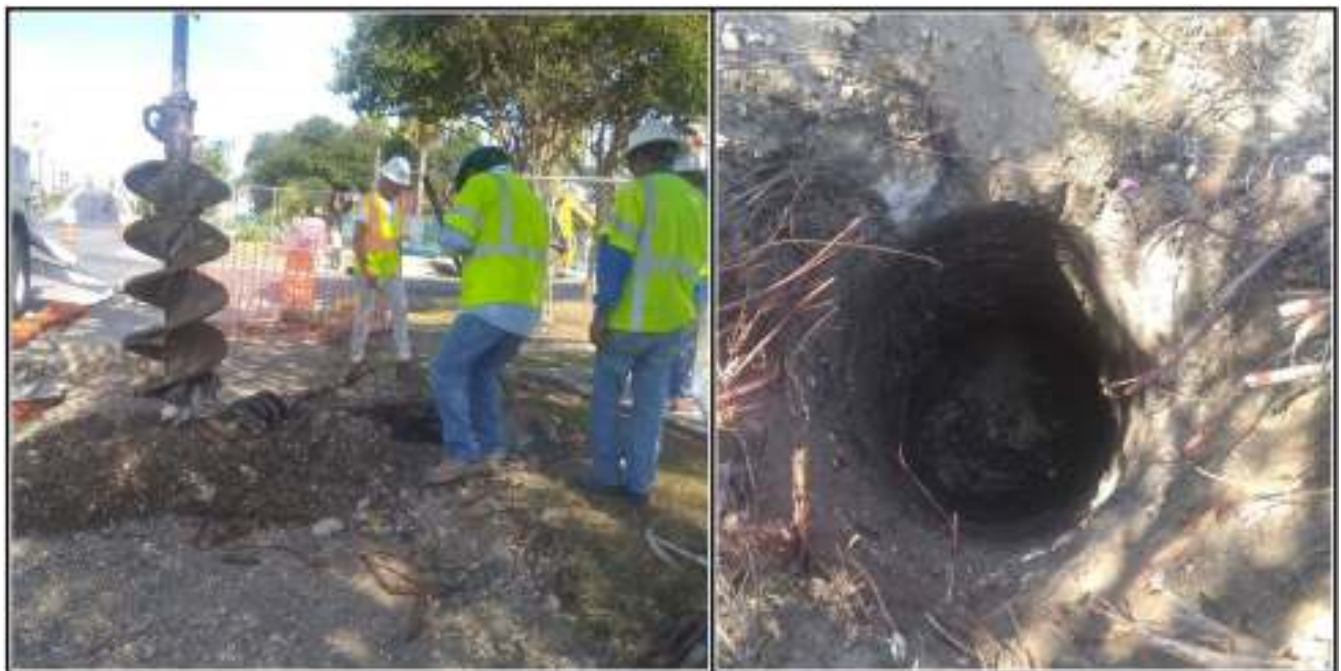
Figure 6-7. Auger excavation at S. Leona and Buena Vista streets (left). The image of the right shows concrete at 152.4 cm (5 ft.) below the surface.
