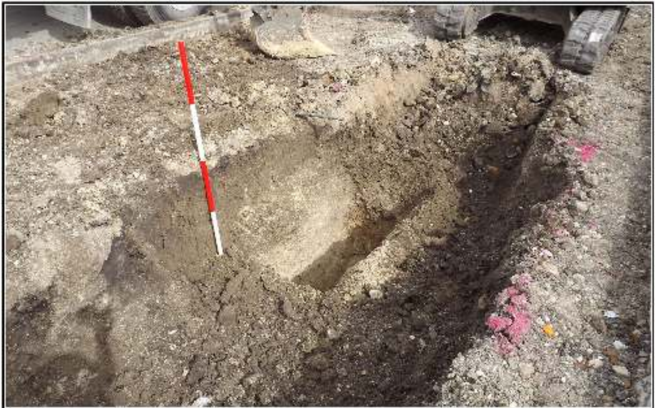
Figure 6-11. Typical pit excavation with deeper drainage pit against the wall and soil profile.
