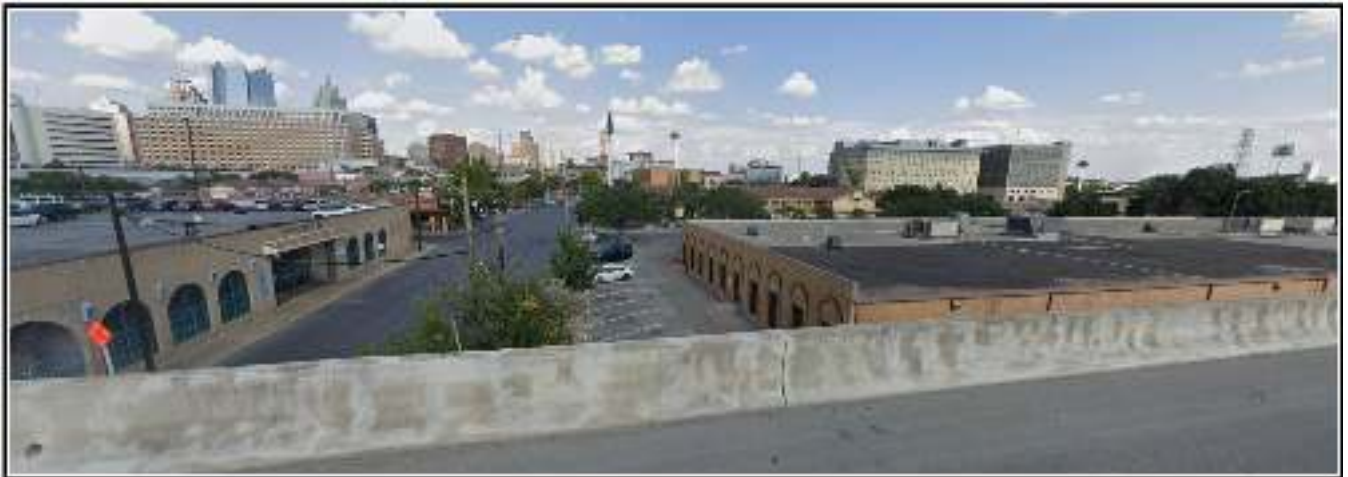
Figure 1-4. View of project area from the S. Pan Am Expressway to the east showing the Farmer's Market Building on the left and an office building on the right (Google Street View, August 2019).
