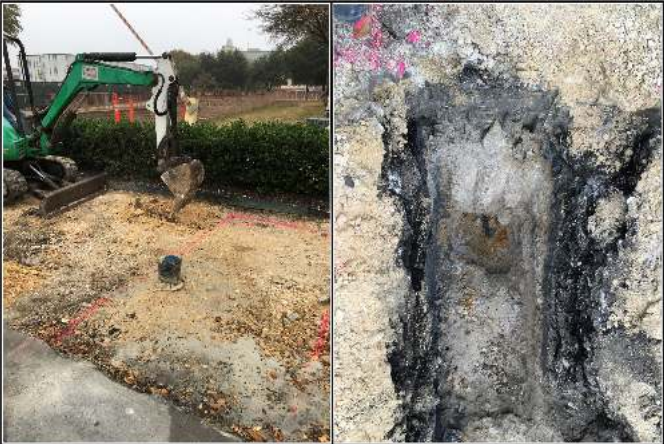
Figure 6-4. Excavation of Trench 3 on the south side of Buena Vista and S. Leona streets (left). The right image shows the trench with asphalt and flowable fill over an existing cast iron pipe.
