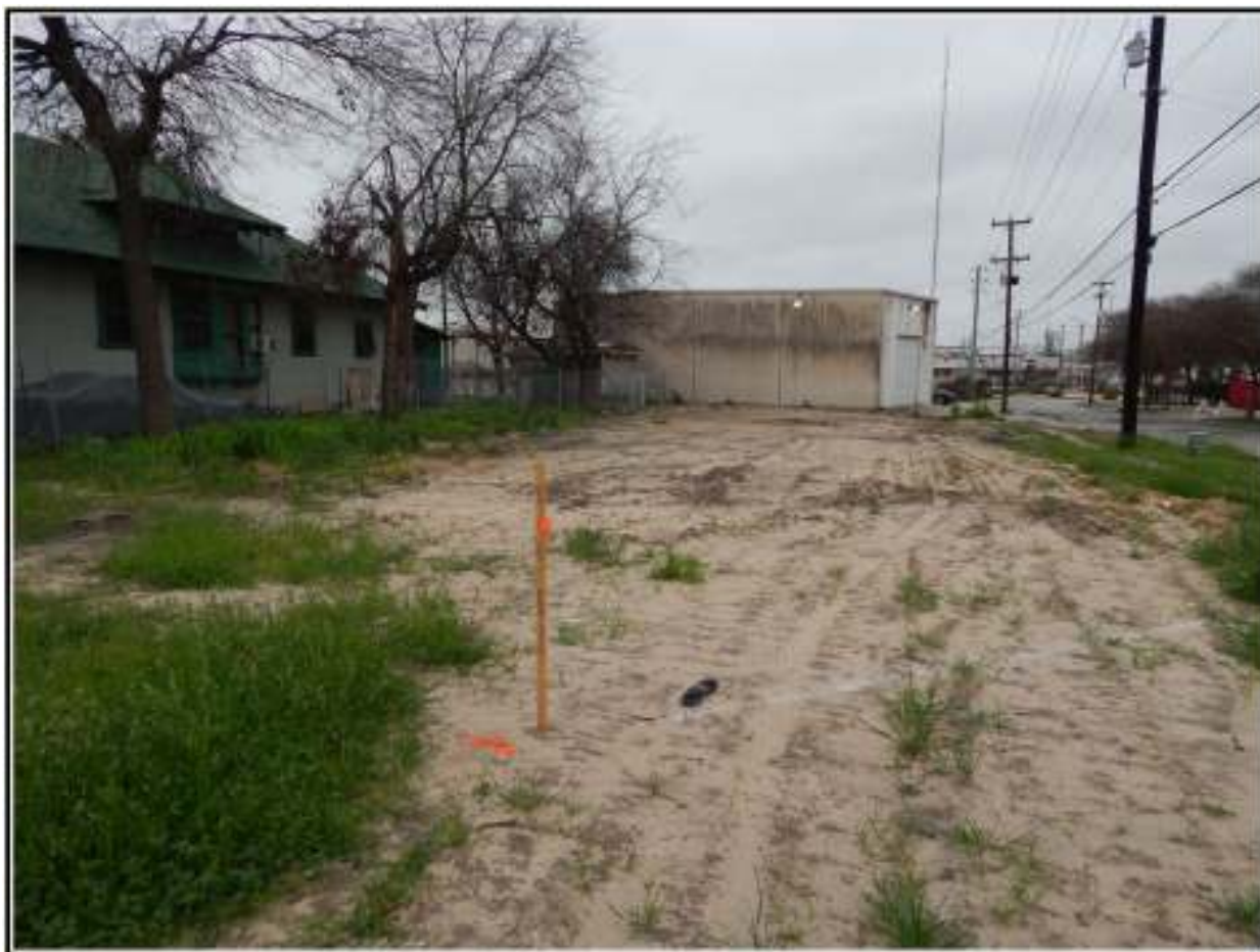
Figure 4-13. Project Area 2, prior to excavation (facing west). Southern property boundary is the chain-link fence with the western boundary defined by the structure and northern boundary inside the utility poles.
