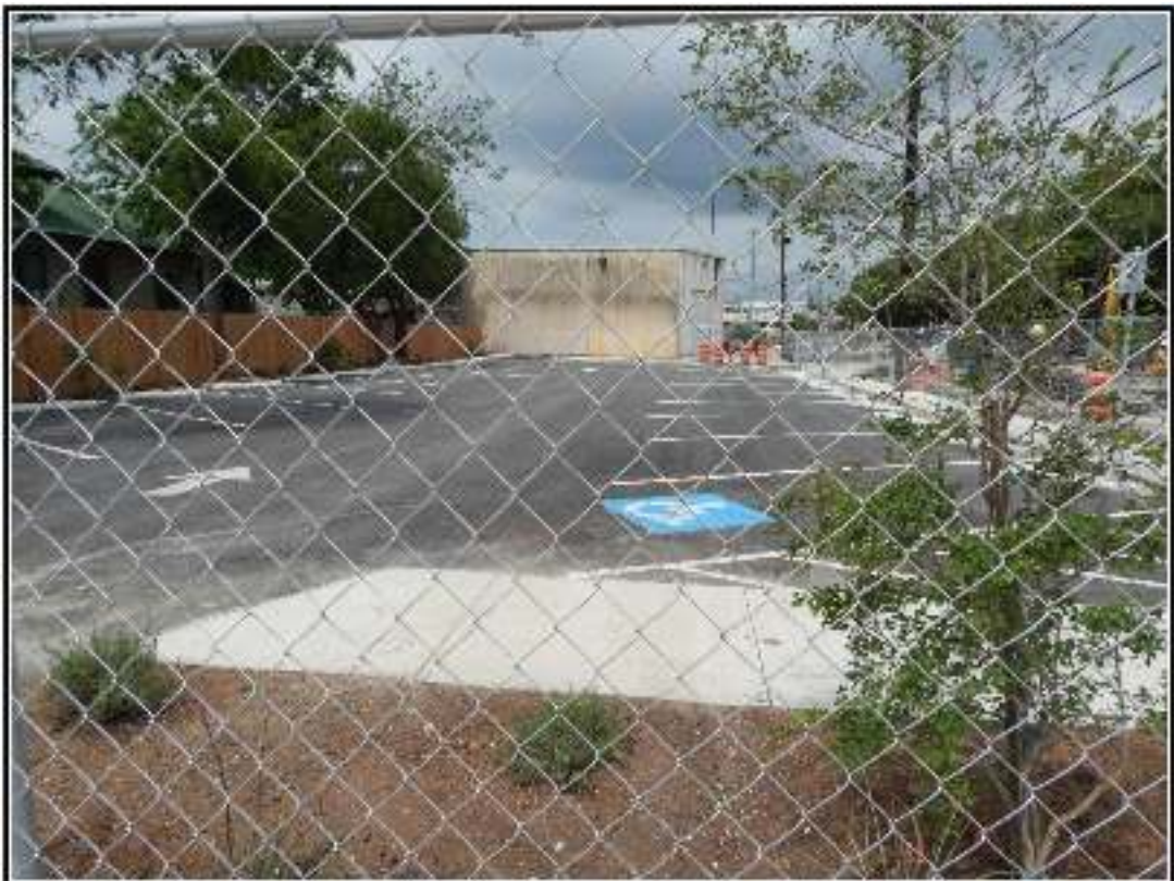
Figure B-2. Project Area 2, looking west.
