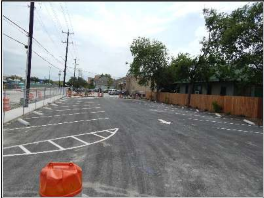
Figure B-1. Project Area 2, looking east.
