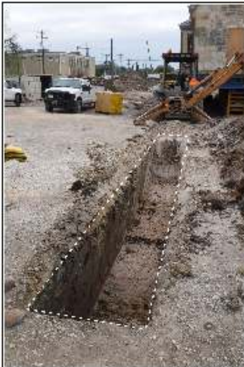
Figure 4-6. Backhoe Trench 4, excavation completed.
