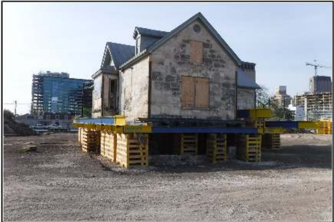
Figure 4-8. View of house raised above original footings.
