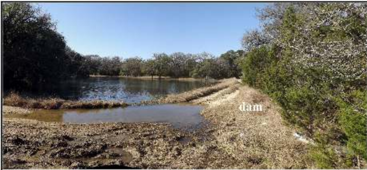
Figure 6-19. A view to the northwest of Feature 3.
