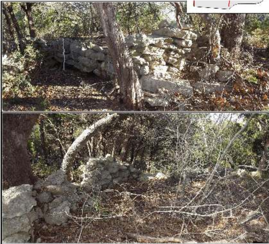
Figure 7-33. Views of 41BX2306 Feature 2. The top image is an exterior view orientated to the northwest. The bottom image is an interior view to the southeast.
