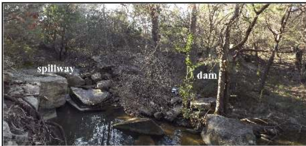
Figure 6-18. A view to the northwest of Feature 2.
