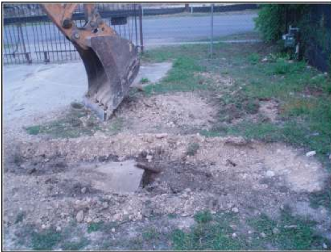
Figure 4-3. Backhoe Trench 1, facing northwest.
