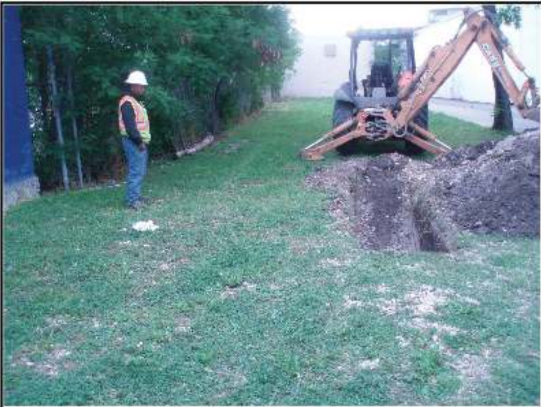
Figure 4-5. Backhoe Trench 3 location, facing southeast.
