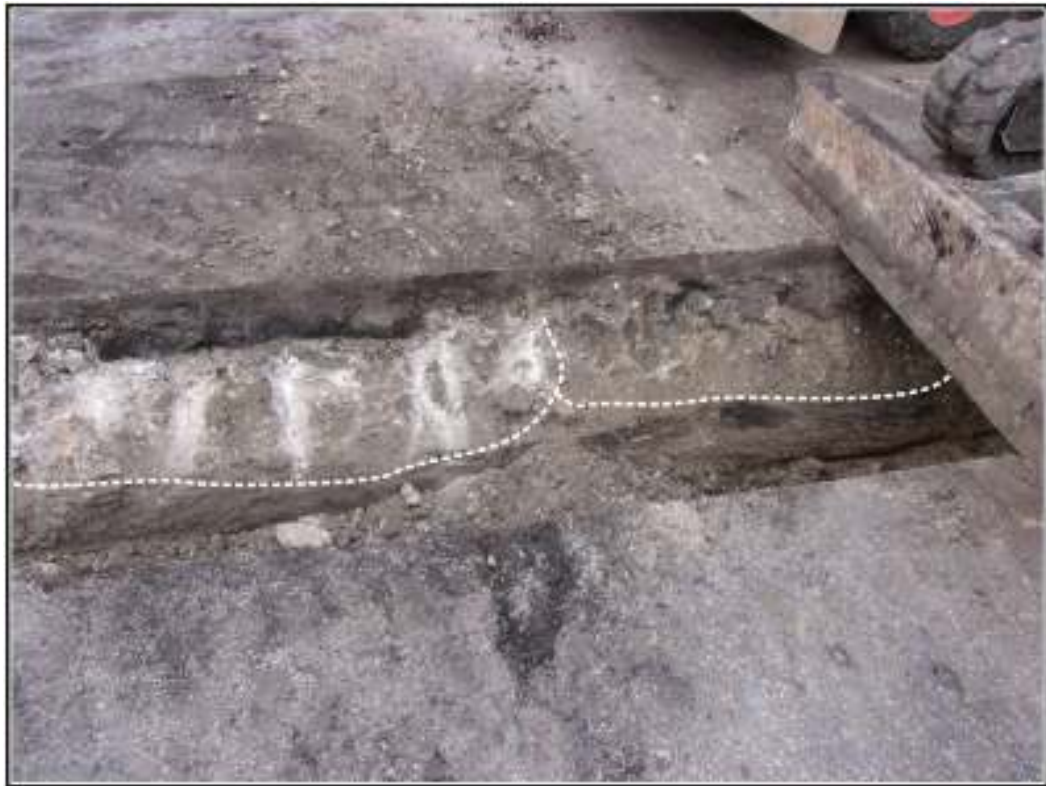
Figure 4-2. Trench profile depicting previous road layers and road base associated with multiple street modifications. Dotted white lines to the left show old concrete, to the right show layer of road base.
