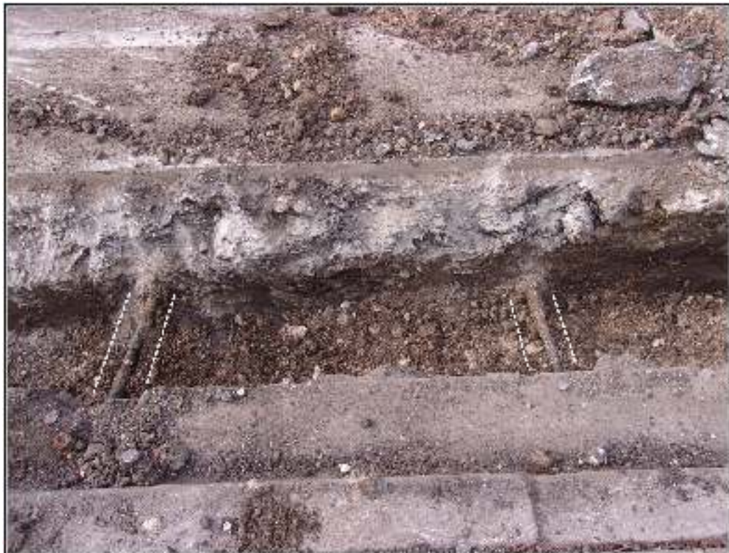
Figure 4-3. Utility pipes within monitored trench. Dotted white lines illustrate pipes.
