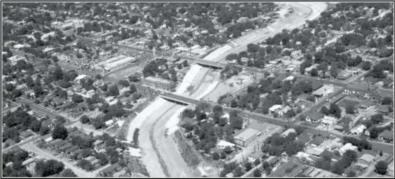
Figure 2-10. Aerial photograph (dating to the 1970s) that shows the channelized Alazán Creek (SARA 2011:9).
