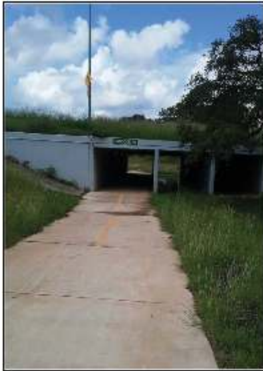
Figure 4-2. Existing trail that crosses west under Babcock Road.
