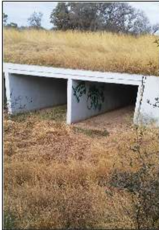
Figure 4-7. Maverick Creek and culvert west of ST 3, facing west.
