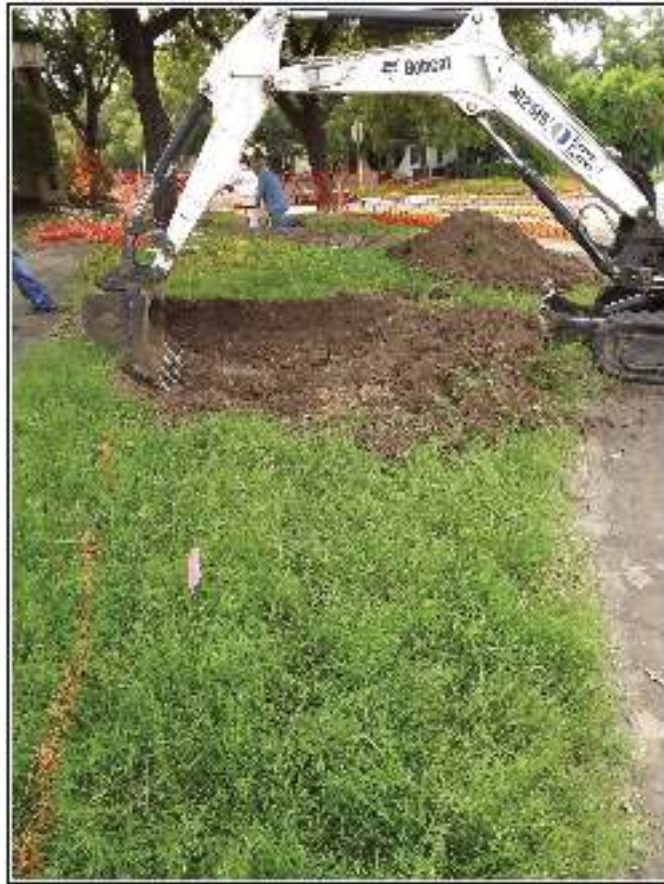
Figure 4-3. A view to the southeast of the excavation for kiosk foundation.
