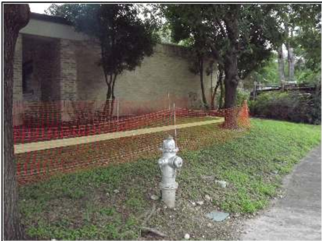
Figure 1-3. View to the northeast of proposed trench (highlighted area) with tie-in to the visitor's center.
