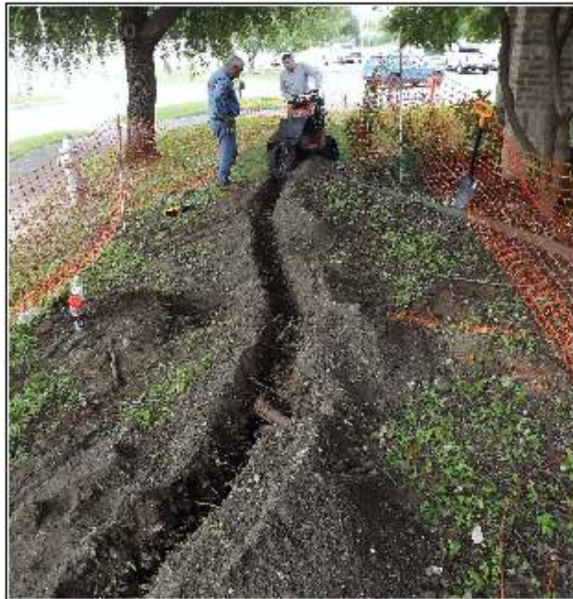
Figure 4-1. View to the west of trench excavation adjacent to visitor's center.
