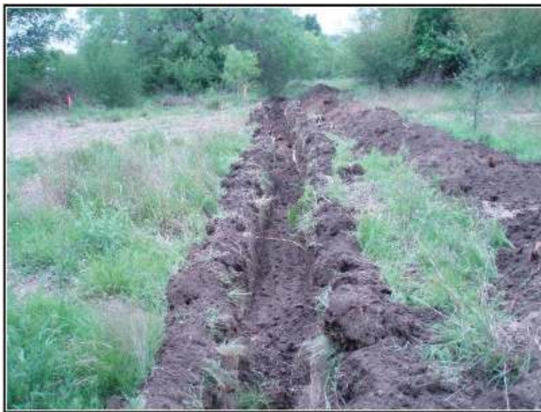
Figure 4-9. Partially excavated backhoe trench along the western perimeter of the site.
