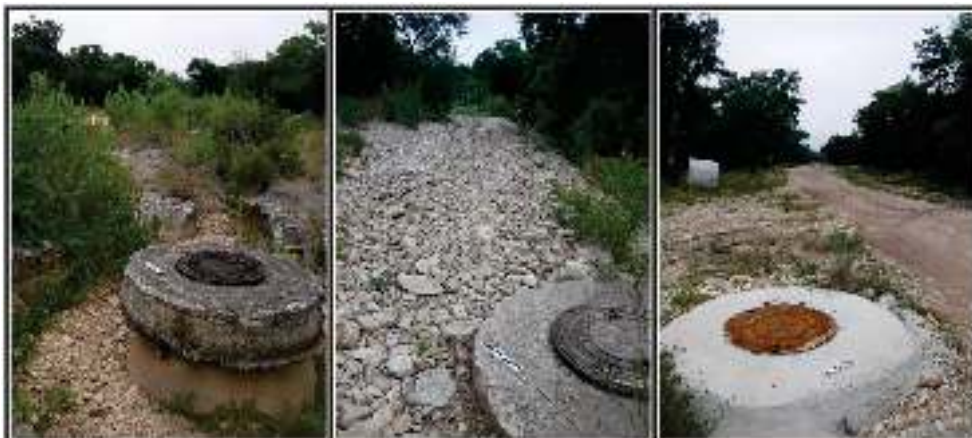
Figure 4-8. Trail following path of sewer line easement from view northeast (left), northeast (center), and northwest (right).
