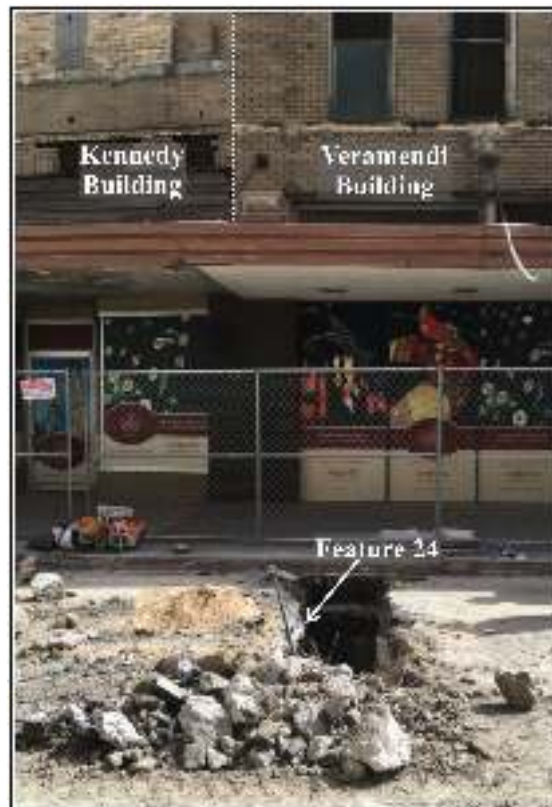
Figure 9-6. Location of Feature 24 in lateral trench in front of Veramendi and Kennedy Buildings.
