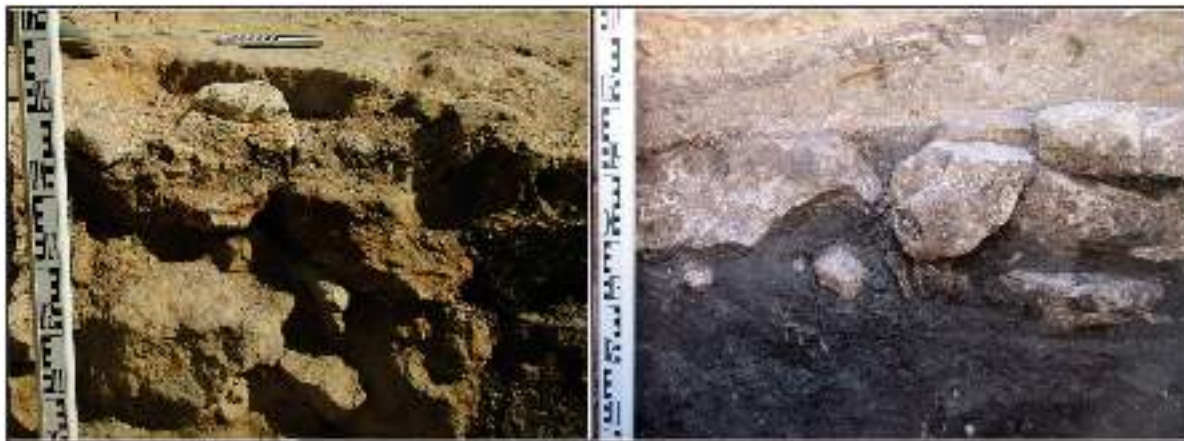
Figure 8-13. Feature 3, wall footing set in caliche/silt slurry, and Feature 9, wall footing set in mud, showing the difference in the construction of the wall alignments.
