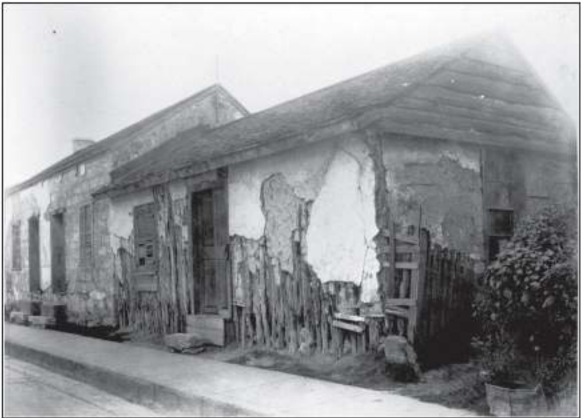
Figure 4-6. A caliche-block house, less its plastering, is shown on the left with a palisado (vertical logs placed in a trench) style house on the right on Laredo Street, San Antonio, circa 1920-1929 (UTSA General Photograph Collection 101-0057). The image also appears in Fisher 1996.
