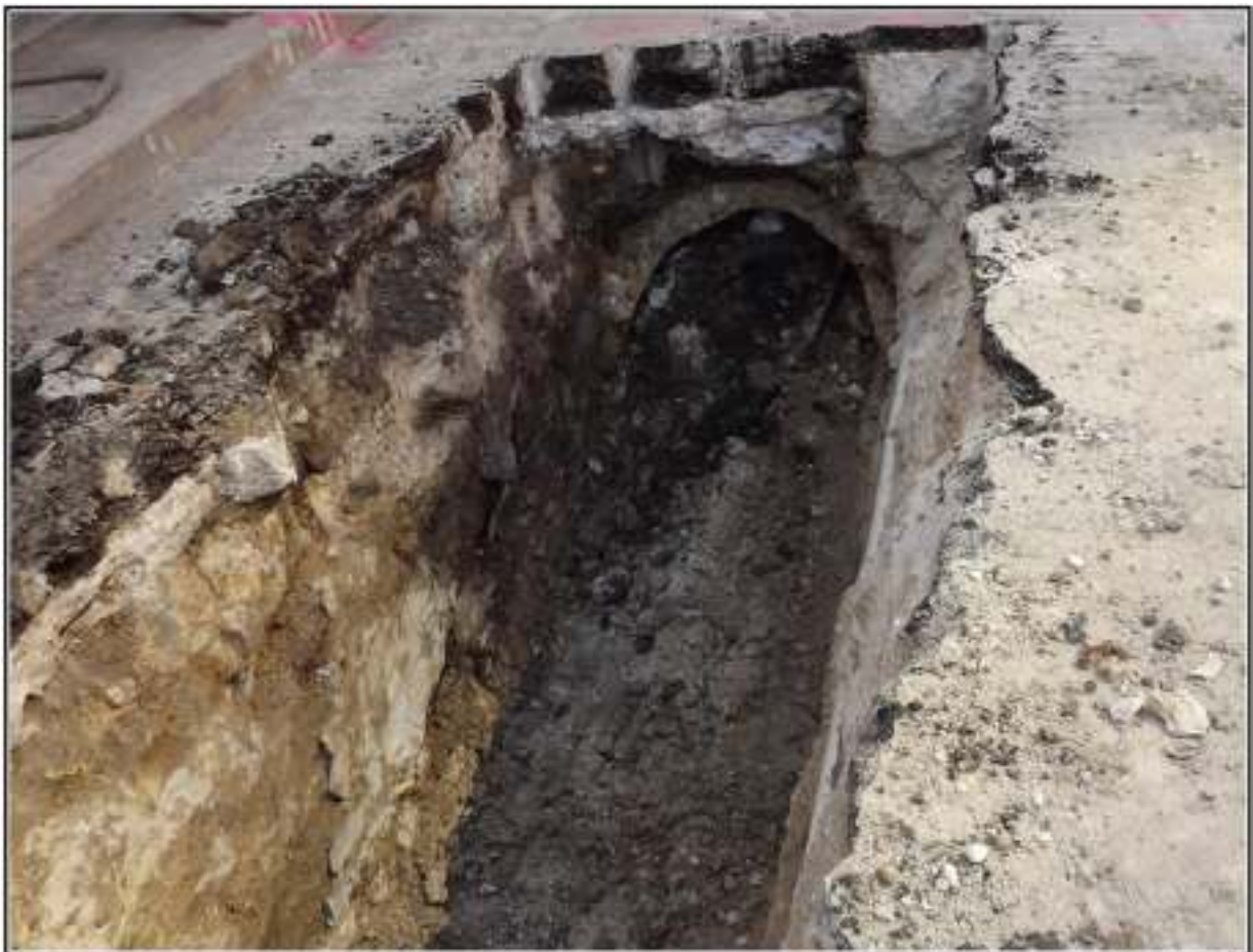
Figure 7-32. East wall of the acequia with a formed-in-place storm pipe.
