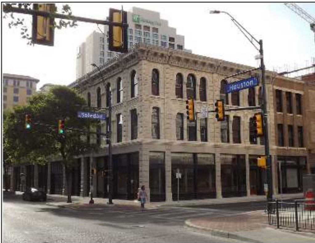
Figure 5-34. The Soledad Block after removal of slipcover and restoration.
