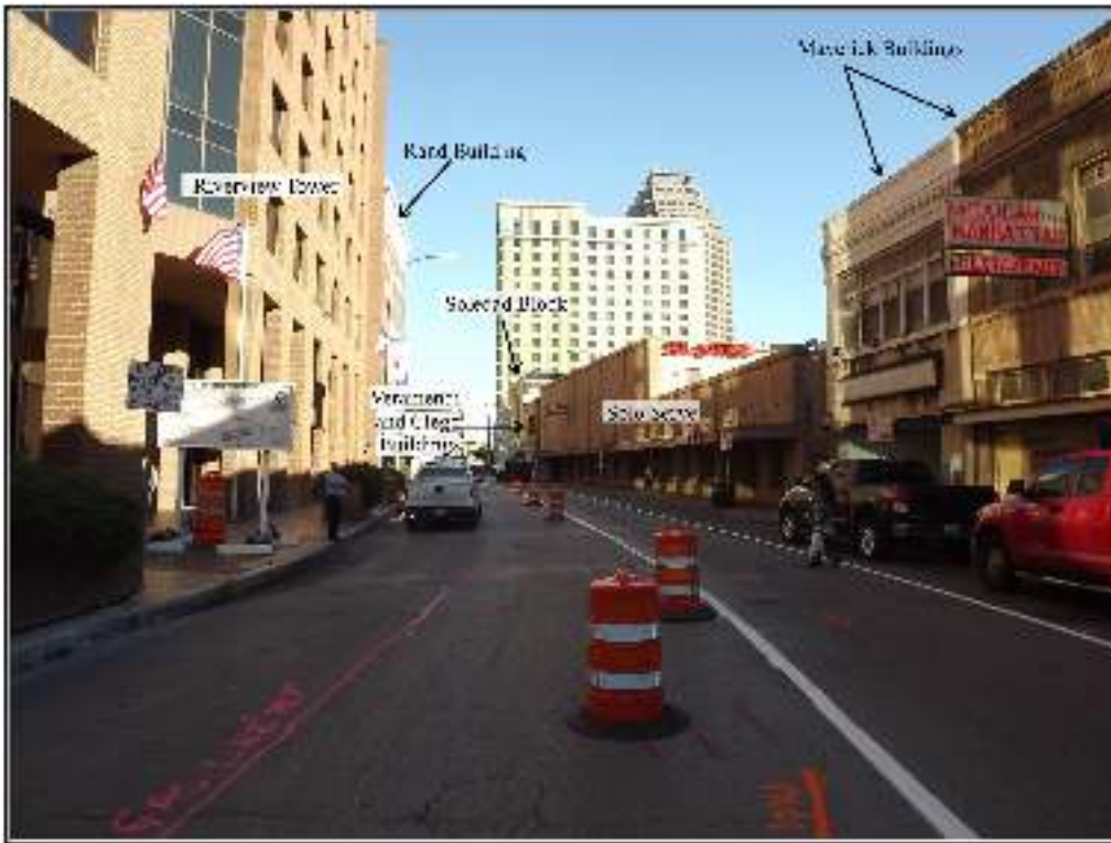
Figure 2-1. View to the north of the 100 block of Soledad Street in October 2016. The parking garage between the Riverview Tower and the Rand Building on the left side of the image is obscured. A large portion of Riverview Tower is leased to the COSA.
