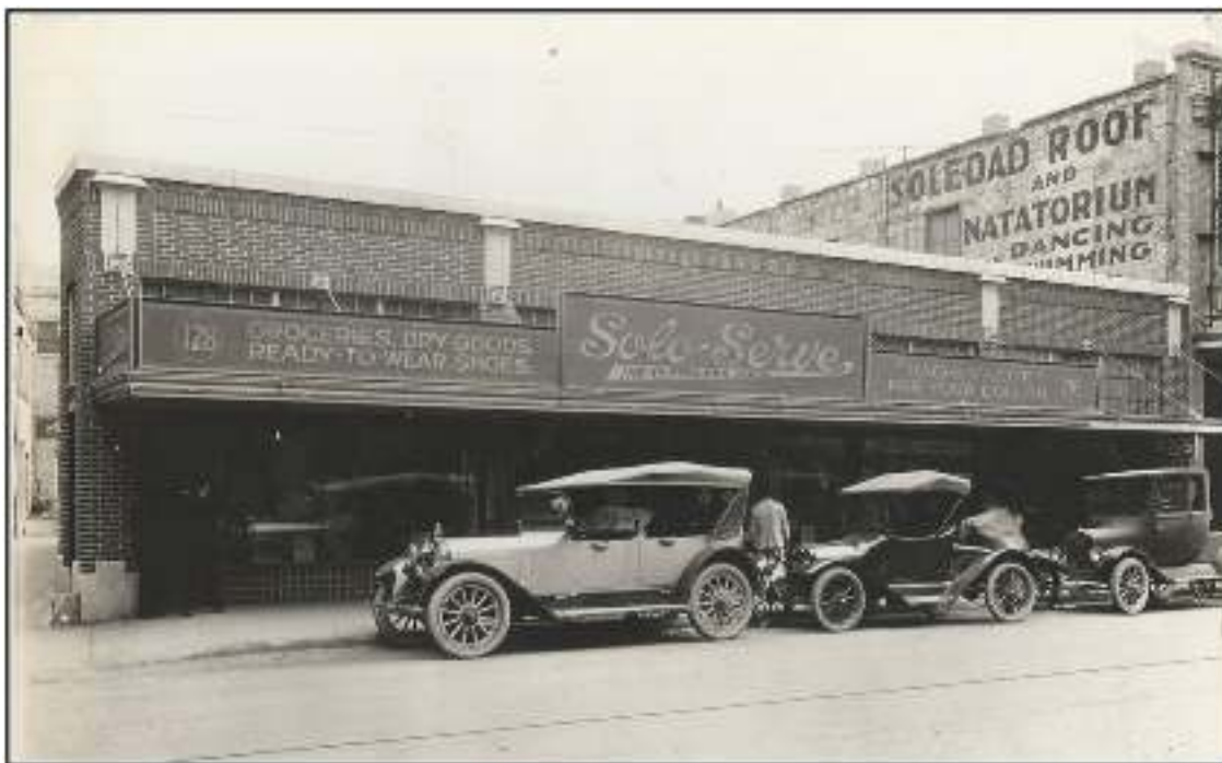
Figure 5-24. Solo Serve Building in 1922 (Image courtesy of Irene Dunn).
