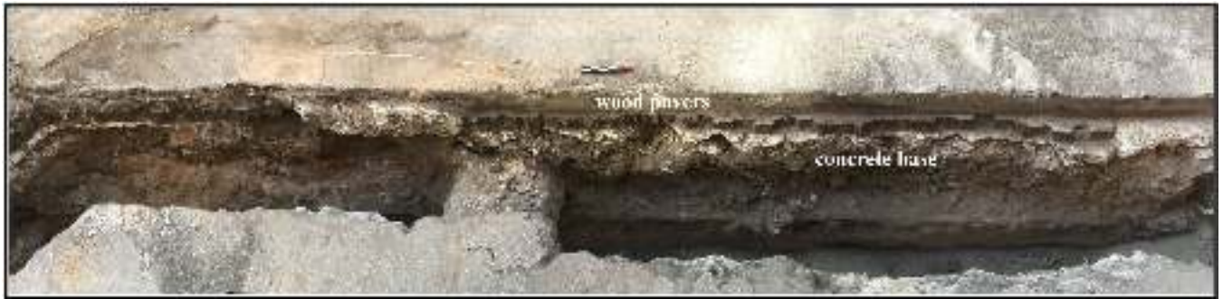
Figure 7-17. Cross section of Feature 22 (wood pavers) and concrete base on Main Avenue.
