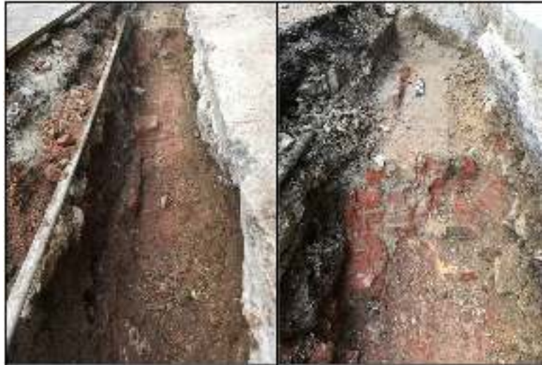
Figure 7-21. Feature 23, foundation remnant of 41BX2203. The image on the right shows the wythe brick construction of the feature.
