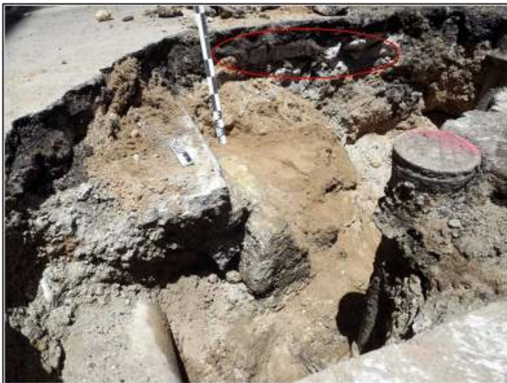
Figure 7-26. Photo shows the east wall of the acequia near the south entrance of the Frost Parking Garage. A portion of that wall was removed by past utility construction. The red ellipse delineates wood block pavers (Feature 22).
