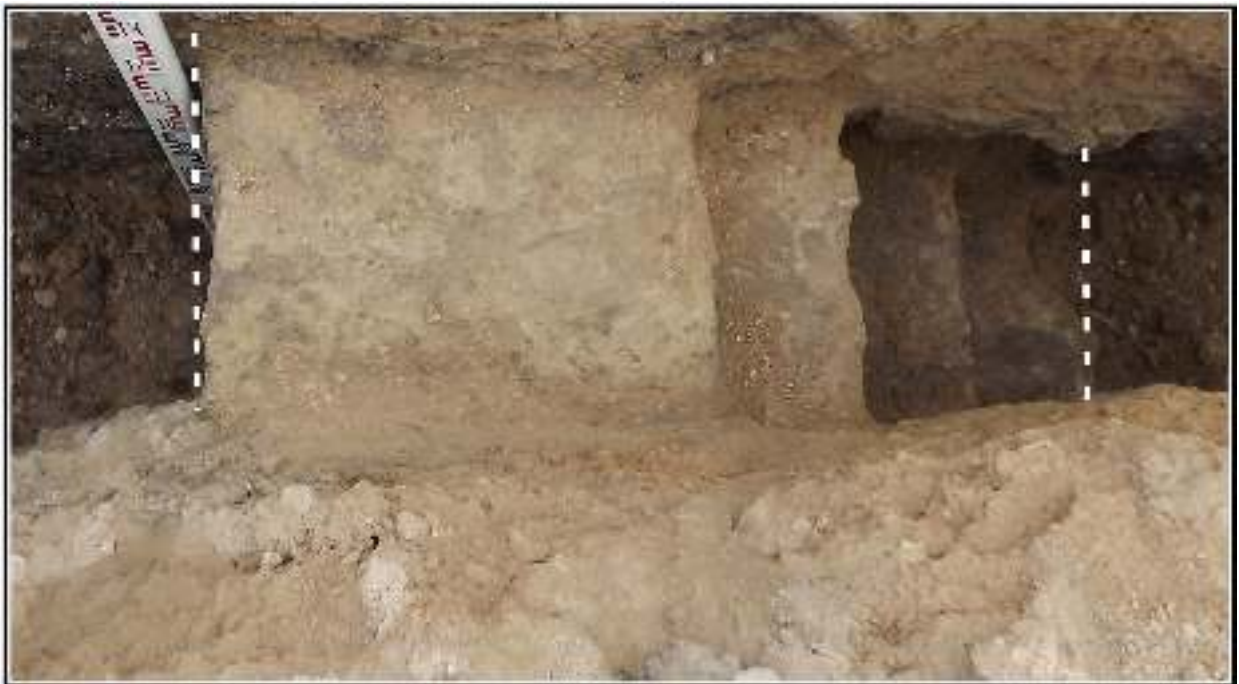
Figure 5-6. Feature 3, east-west wall segment (between white lines), facing west. Scale is metric.
