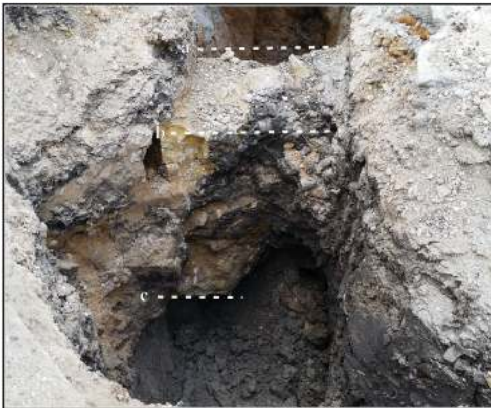
Figure 5-40. Feature 16, north-south wall segment of Alazán Ditch, facing northwest. Horizontal extent of feature shown between lines a and b. Vertical extent of feature shown between lines b and c.
