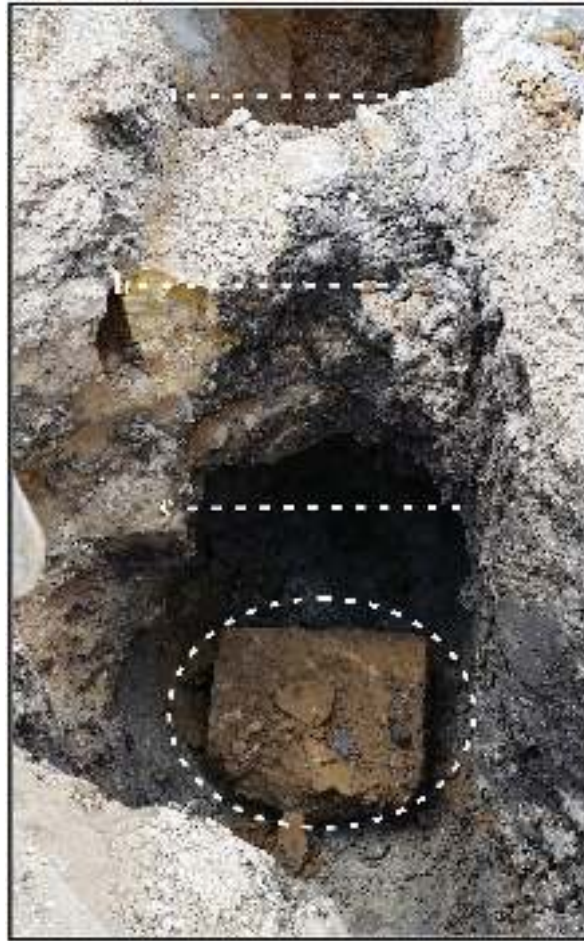
Figure 5-41. Feature 16, Alazán Ditch (41BX620) wall segment and fallen stone from bottom of the wall (outlined in white), facing northwest. Horizontal extent of feature shown between lines a and b. Vertical extent of feature shown between lines b and c.
