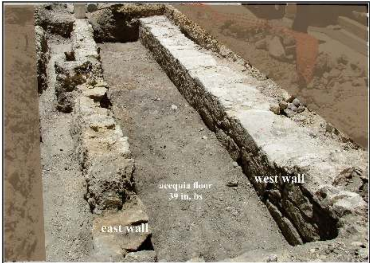
Figure 5-9. Exposed section of the Acequia Madre de Valero (41BX8); note dissimilarities between the walls and the concrete support installed through the east wall at top left (bs=below the surface). Periphery shaded to focus on acequia (view south).
