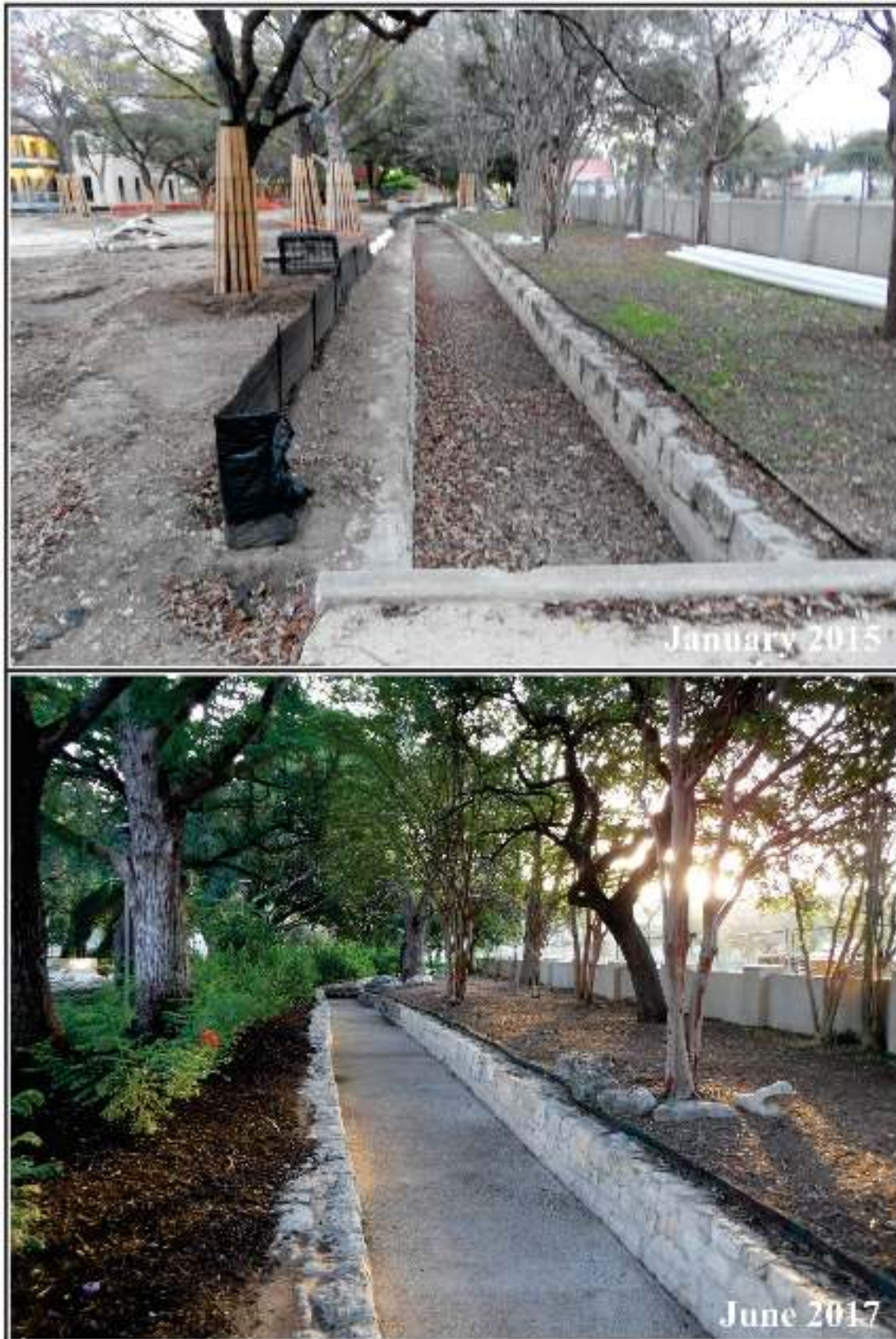
Figure B-10. Reconstructed acequia (view north).
