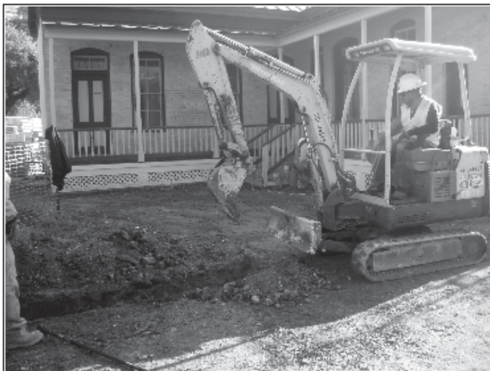
Figure 7-9. Excavations for water lines at the Espinoza House (41BX593).
