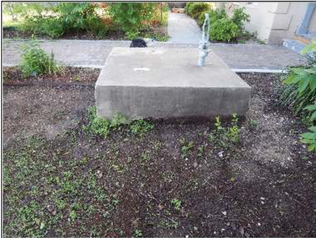
Figure 7-11. Well at the Pereida House (41BX591).
