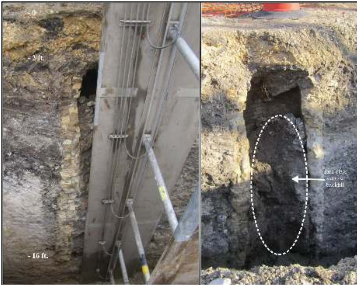
Figure 8-10. Feature 1, manhole at center of Hemisfair Way approximately 80 ft. north of E. César Chávez Boulevard.
