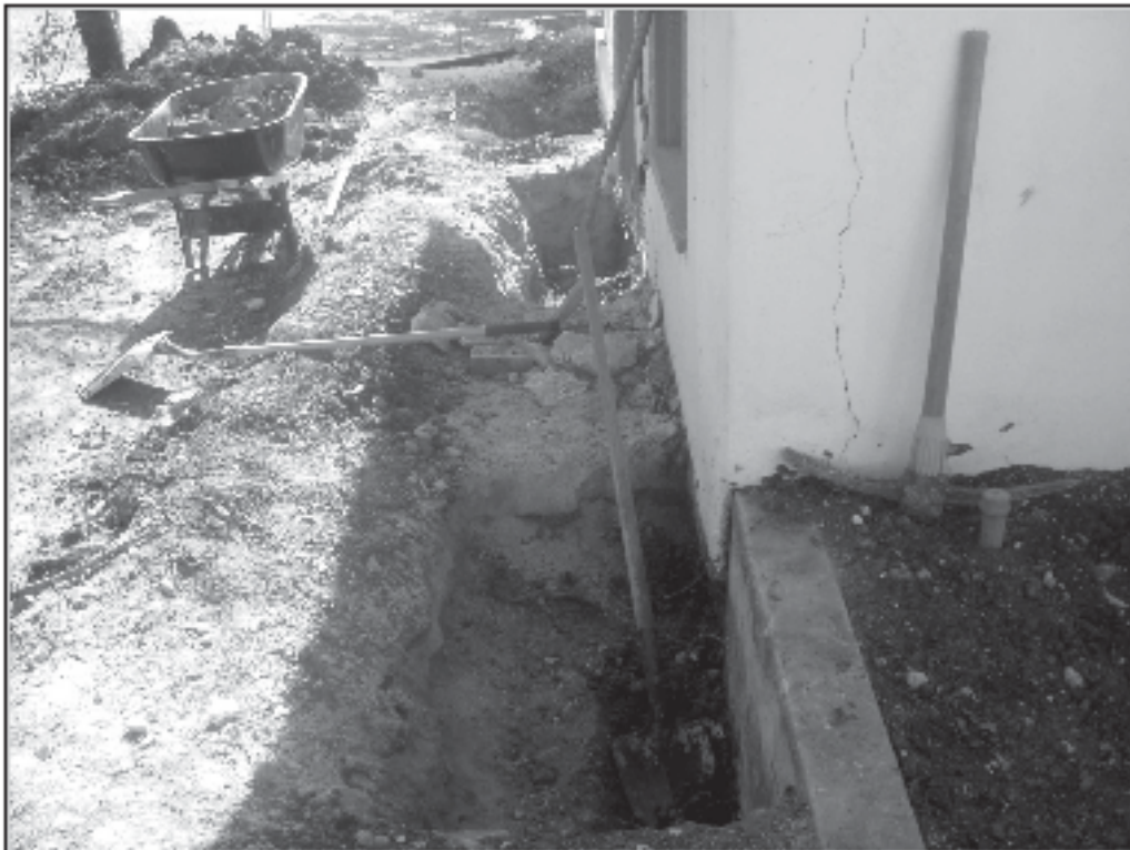
Figure 7-5. Hand excavations on east elevation of the Smith House (41BX589).
