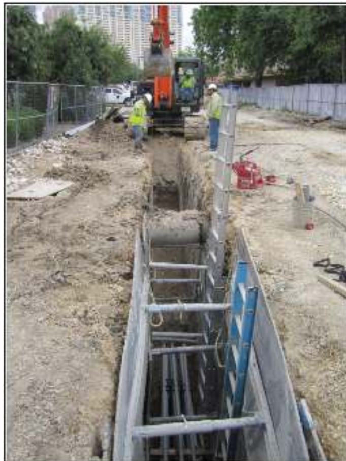
Figure 8-12. Duct bank work along Hemisfair Way (facing north).
