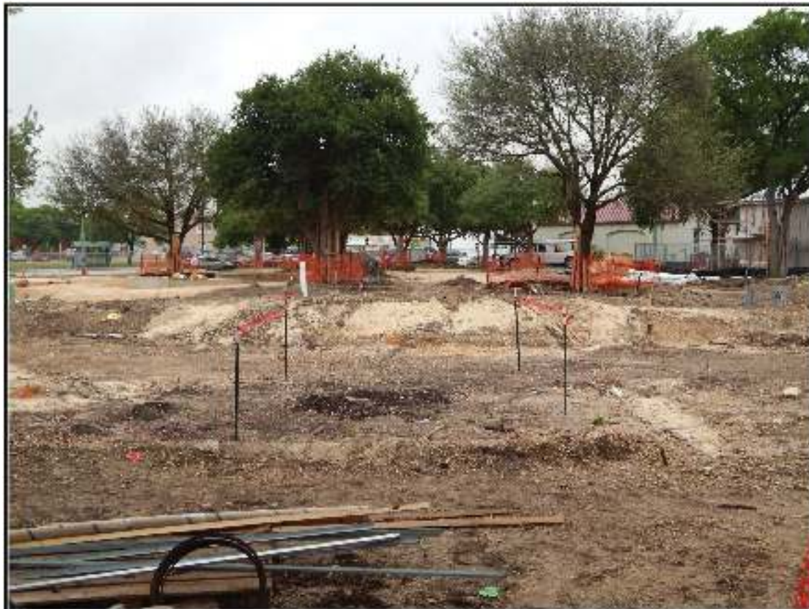
Figure 6-11. T-post barrier marking the pathway of the Acequia Madre de Valero (41BX8).
