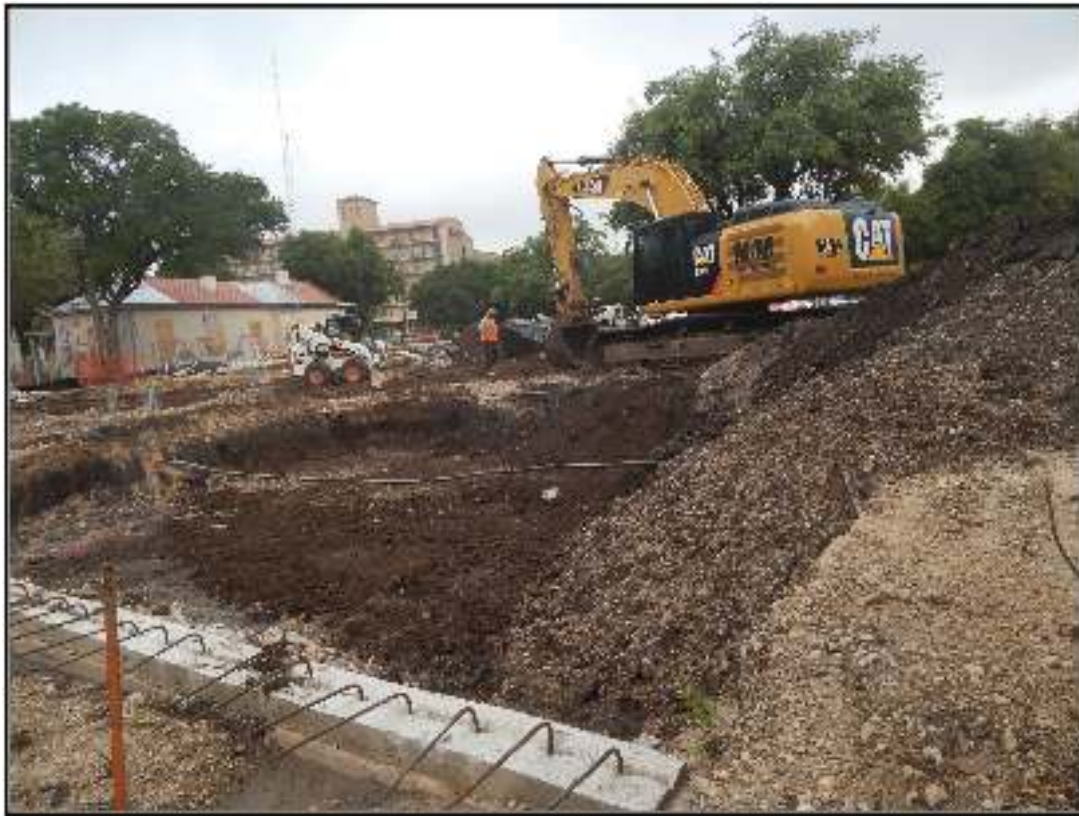
Figure 6-12. Excavation of Splash Pad.
