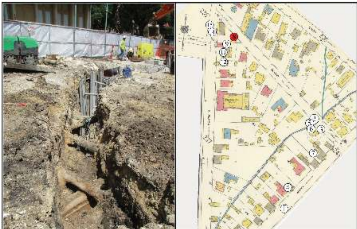
Figure 8-15. Left: duct bank trench north of Feature 8 (likely a privy); note area is heavily disturbed (facing northeast). Right: location of Feature 8 on 1896 Sanborn Fire Insurance Map (Sanborn 1896).
