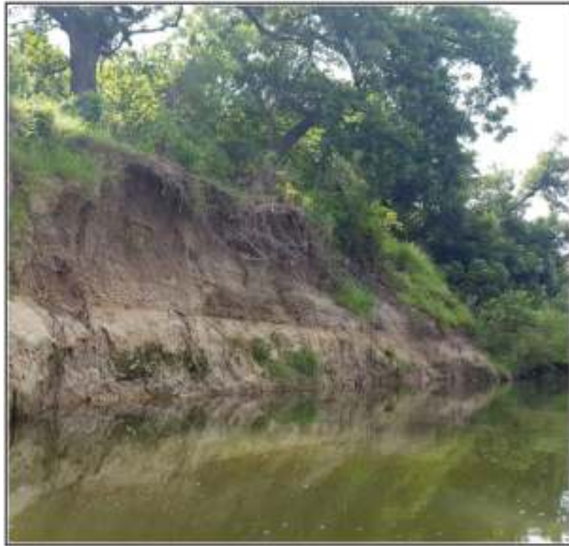
Figure D-4. Shot 311. Below channelized section. Note multiple deposition zones.
