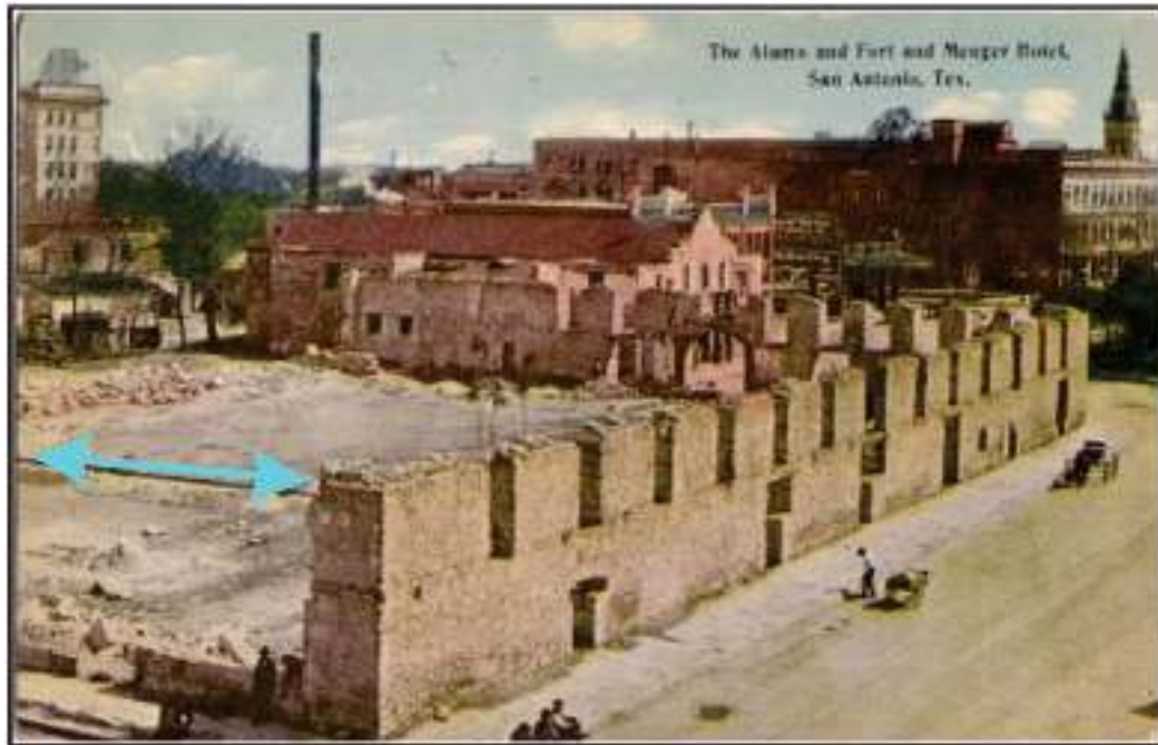
Figure 2-6. The APE following demolition of wooden Hugo & Schmeltzer superstructure, circa 1912. Blue line indicates alignment of north wall of former convento location and location of current wall between the Convento Courtyard and the Calvary Courtyard.
