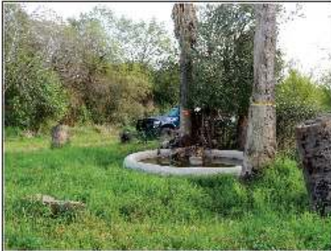
Figure 1-5. Water fountain and gardens immediately east of the bath house and hotel.
