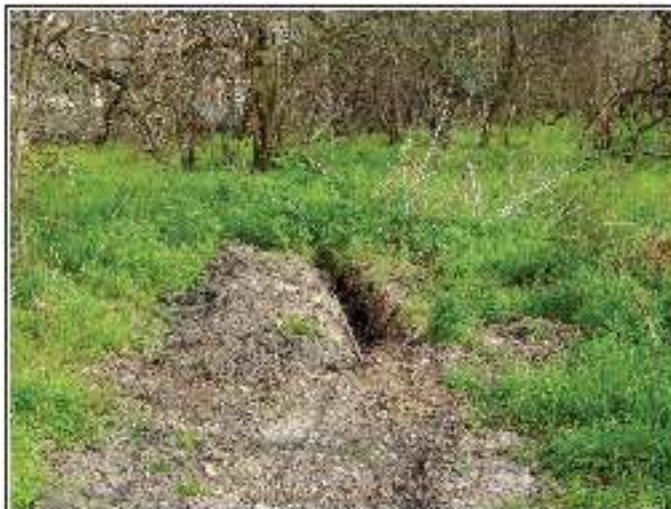
Figure 1-7. Utility trenching in project area.
