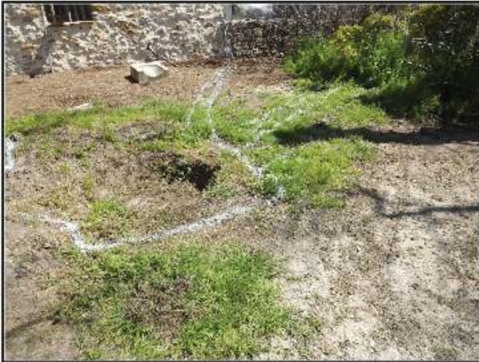
Figure 4-14. Areas excavated for electrical lines for the sump pump.
