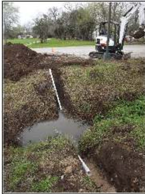
Figure 4-20. View of excavated trench crossing the acequia.
