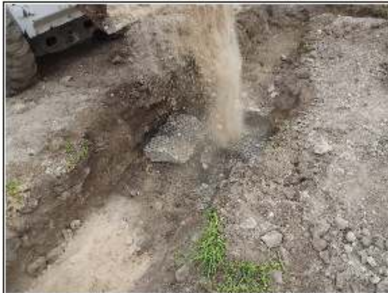
Figure 4-21. Backfilling with sand of wall feature; note plastic webbing.
