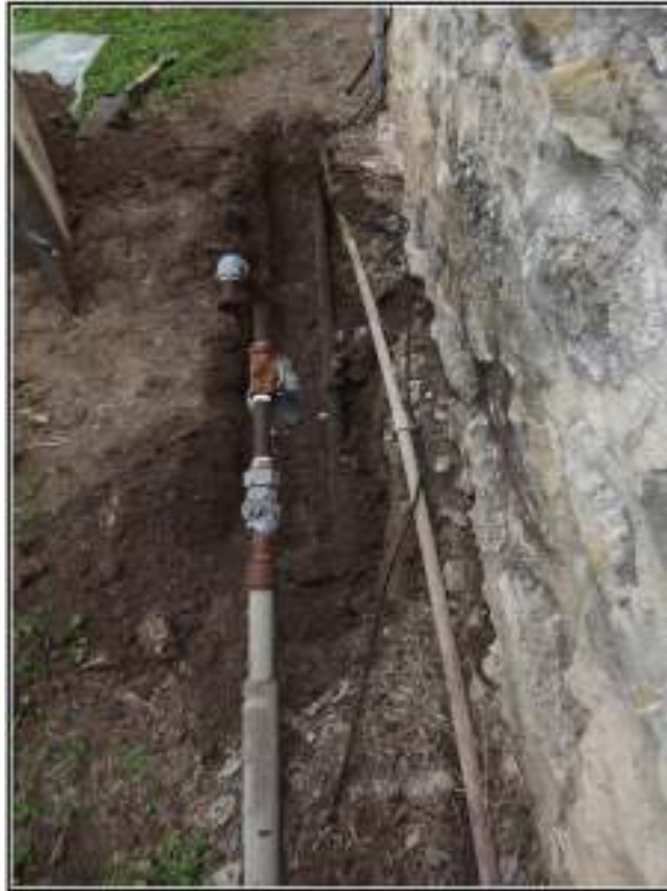
Figure 4-9. Excavation for the water valve box replacement.
