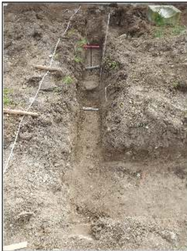
Figure 4-18. View of trench coming from the sacristy showing in situ flagstone, Feature 4, underneath the gas line and probed area of subsurface floor or wall.
