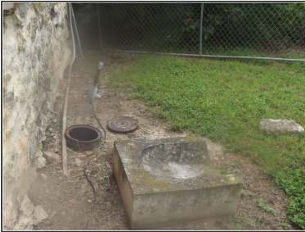
Figure 4-8. Water valve box prior to excavation and replacement.
