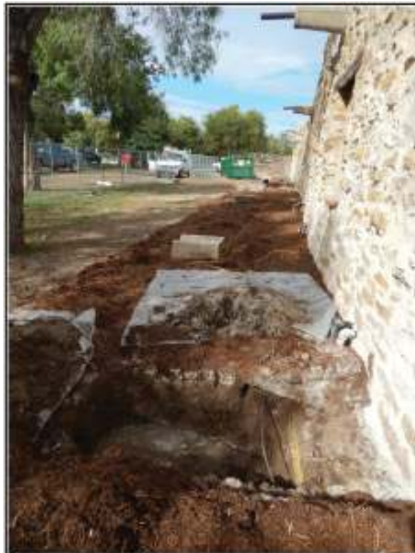
Figure 4-10. Excavations associated with sewage blockage.
