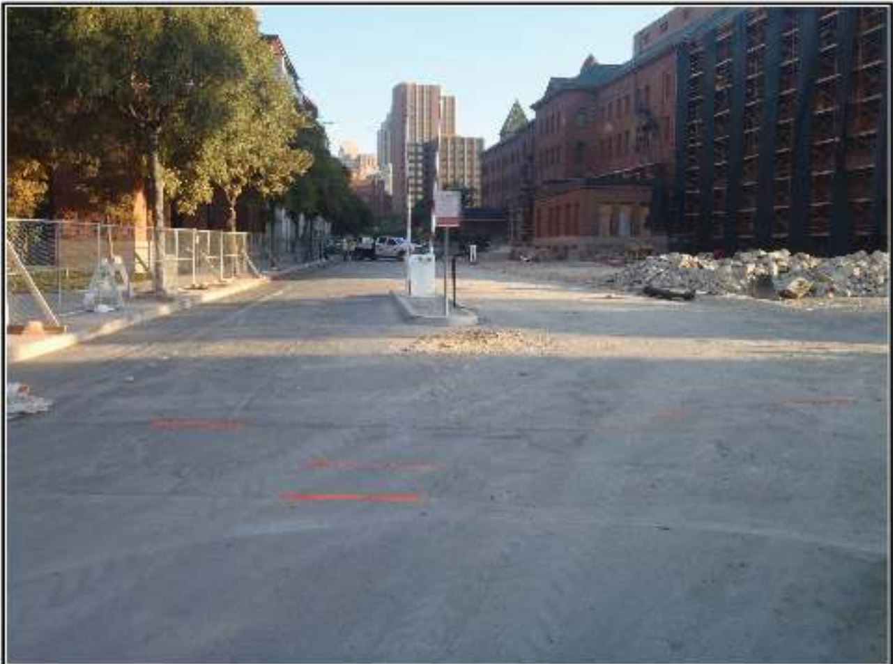
Figure 4-1. Southern portion of Section 1 (facing north).
