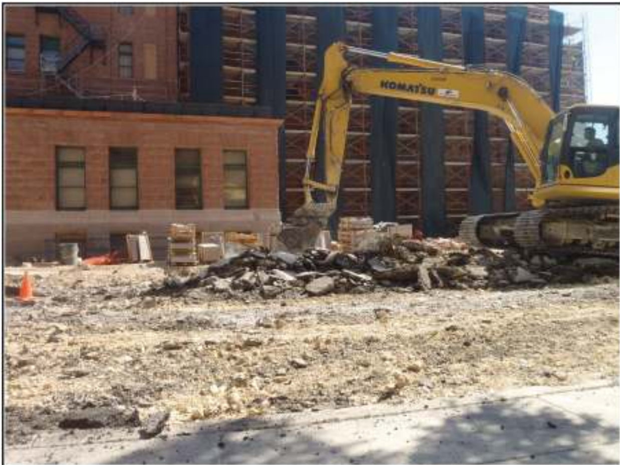
Figure 4-2. Removal of asphalt of Section 2 (facing east).
