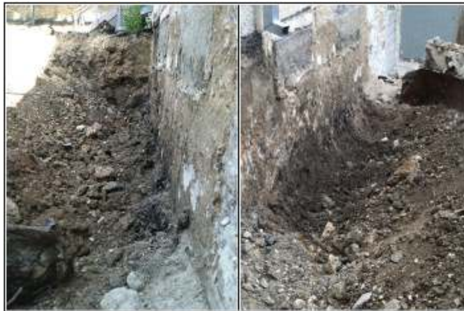
Figure 7-2. Photos of Trench 1, looking north (left) and south (right). Note dark soil at trench base and wall repairs.
