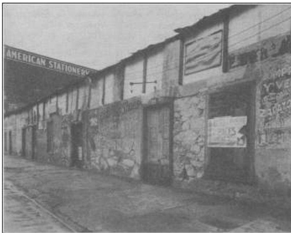
Figure 4-8. The Spanish Governor's Palace prior to reconstruction. North wall of the Plaza de Armas Buildings is visible in the background. Photo ca. 1929 (Hafertepe 2003).
