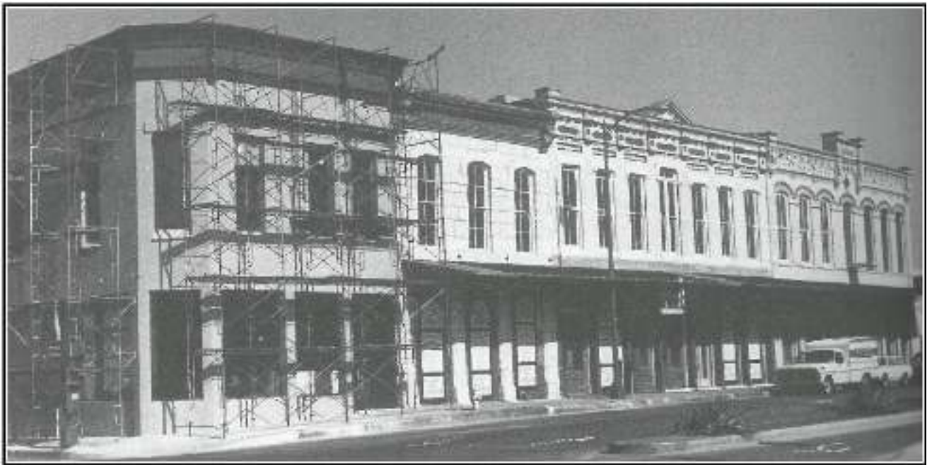
Figure 4-12. The Plaza de Armas Buildings under rehabilitation, ca. 1979-1980 (image from Fisher's Saving San Antonio [1996:380]).
