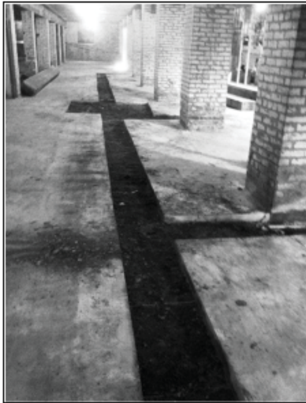
Figure 7-5. Photo of cut in basement floor of Building 1. View is to the east, toward the area of sump (see Figure 7-4). Photo courtesy of Kay Hindes, Office of Historic Preservation, City of San Antonio.
