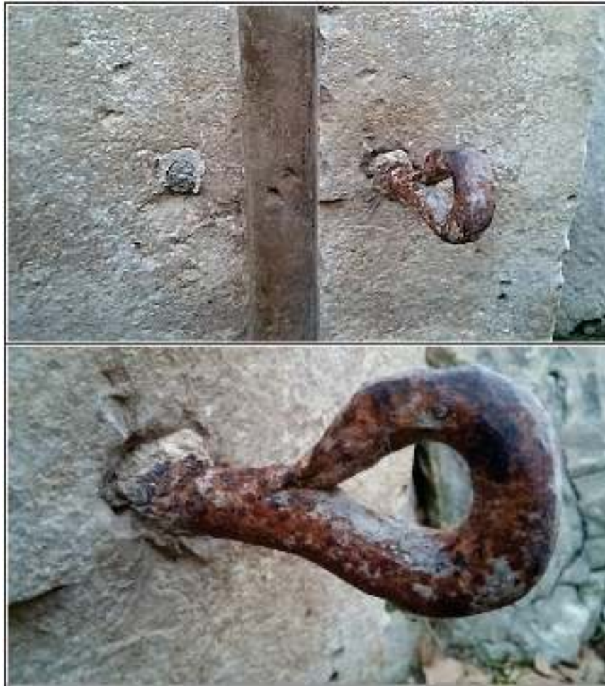
Figure 5-7. Hand-wrought eye-bolt on lower west wall of headgate (top); close-up of eye-bolt (bottom).
