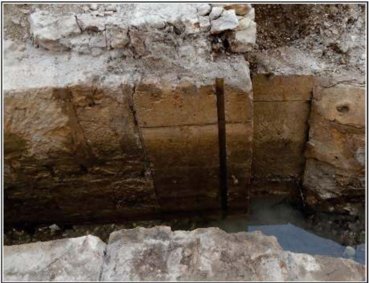
Figure 5-6. West side of headgate exhibiting carved headgate groove and lower eye-bolt.
