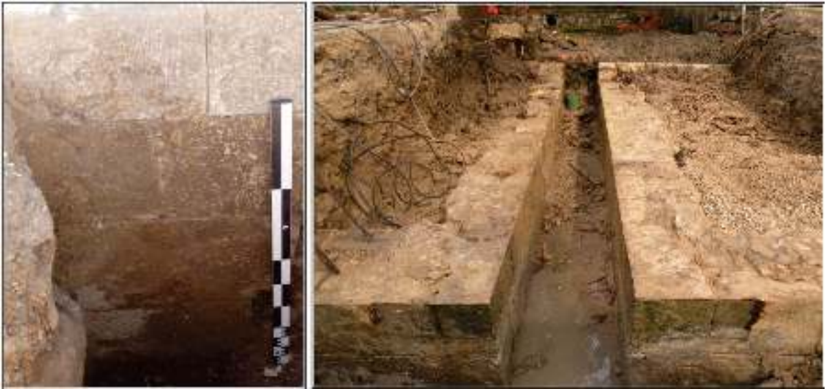
Figure 5-5. Upper Labor Headgate wall (left) and CSA Tannery Sluice walls (right). Comparison of Upper Labor Headgate ashlars to CSA Tannery sluice from Lot 9 exhibiting similar construction. CSA Tannery photograph courtesy of H. Ray Smith and San Jacinto Materials.
