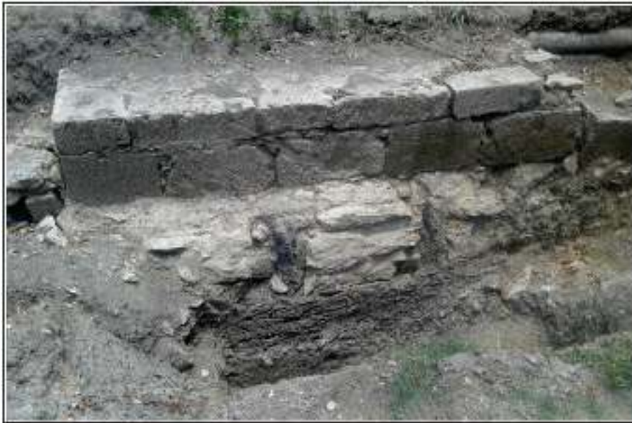
Figure 5-20. Spanish Colonial alignment with vertical wood posts and planking, north end of dam.
