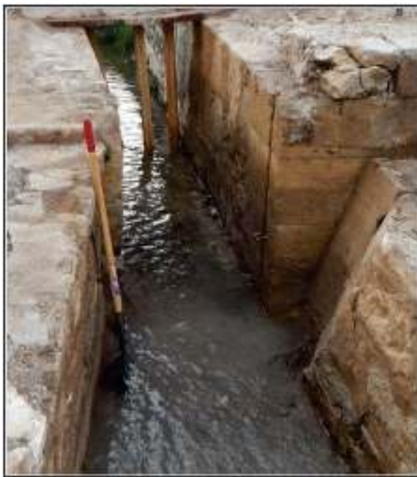
Figure 5-8. Headgate and fore channel of Upper Labor Acequia after removal of concrete slabs.
