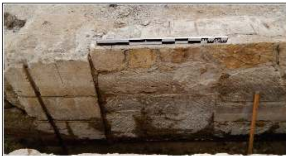
Figure 5-11. Lower channel wall (east) showing whole block construction.
