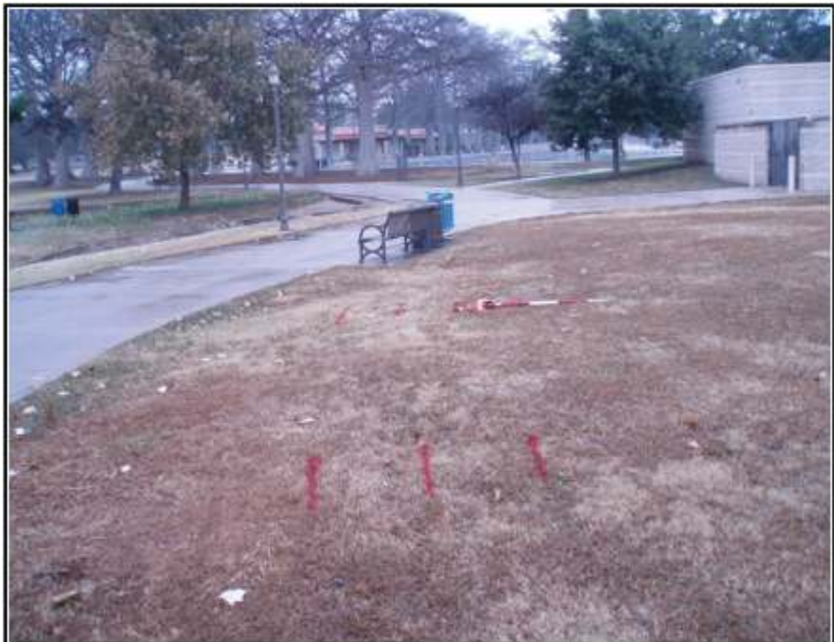
Figure 9-5. Utility lines identified by red paint to the east of the southern sidewalk exit.
