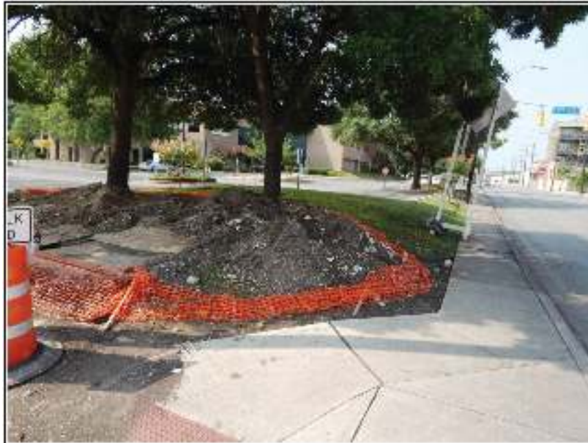
Figure 1-2. Photo of AT&T excavation (facing south).
