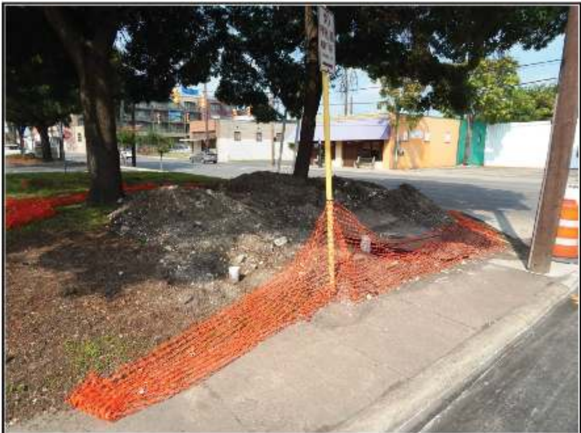
Figure 1-1. Photo of AT&T excavation (facing west).
