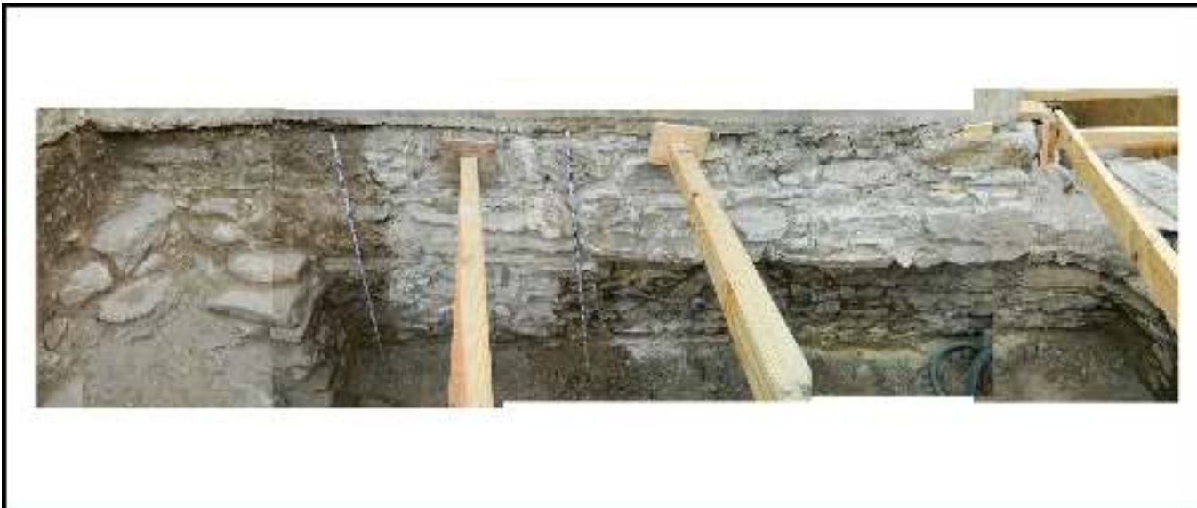
Figure A3-4. The foundation of the north wall of the church.
