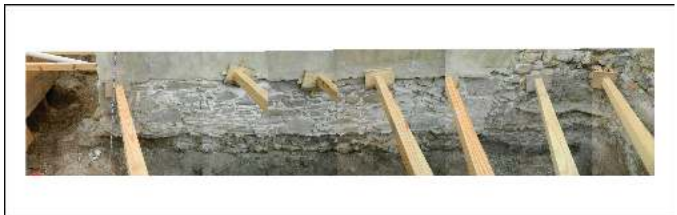
Figure A3-7. The foundation of the south wall of the church.
