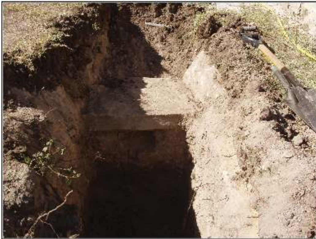
Figure 5-13. Wall uncovered in Backhoe Trench 2.
