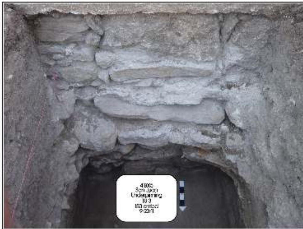
Figure 5-4. Church wall foundation in Test Unit 3.
