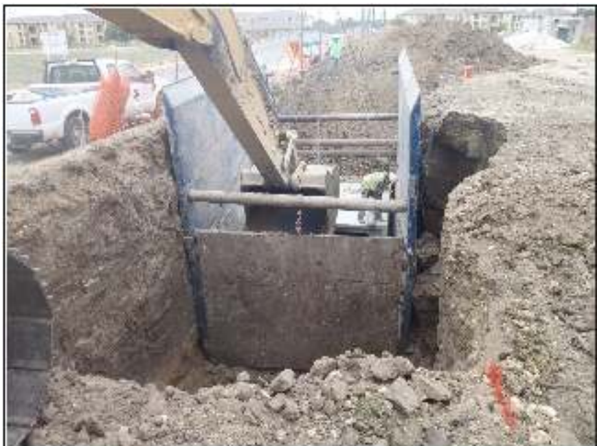
Figure 7-3. Excavator moving the exterior drainage pipe shoring unit.
