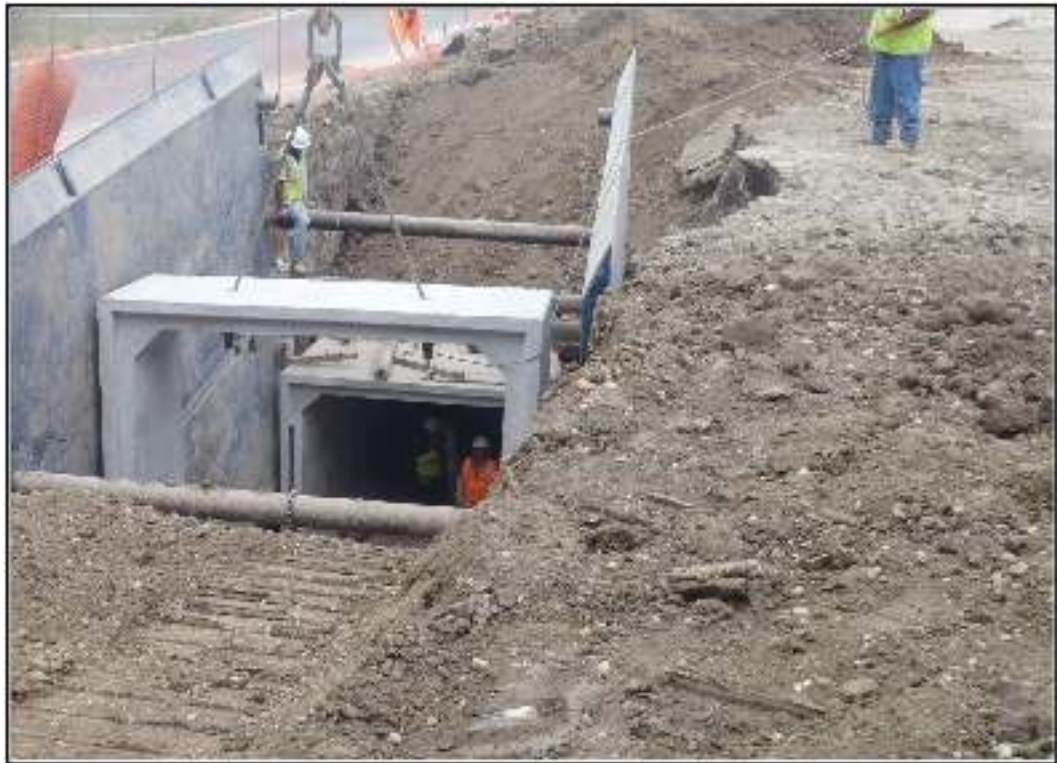
Figure 7-4. Final placement of drainage pipe.
