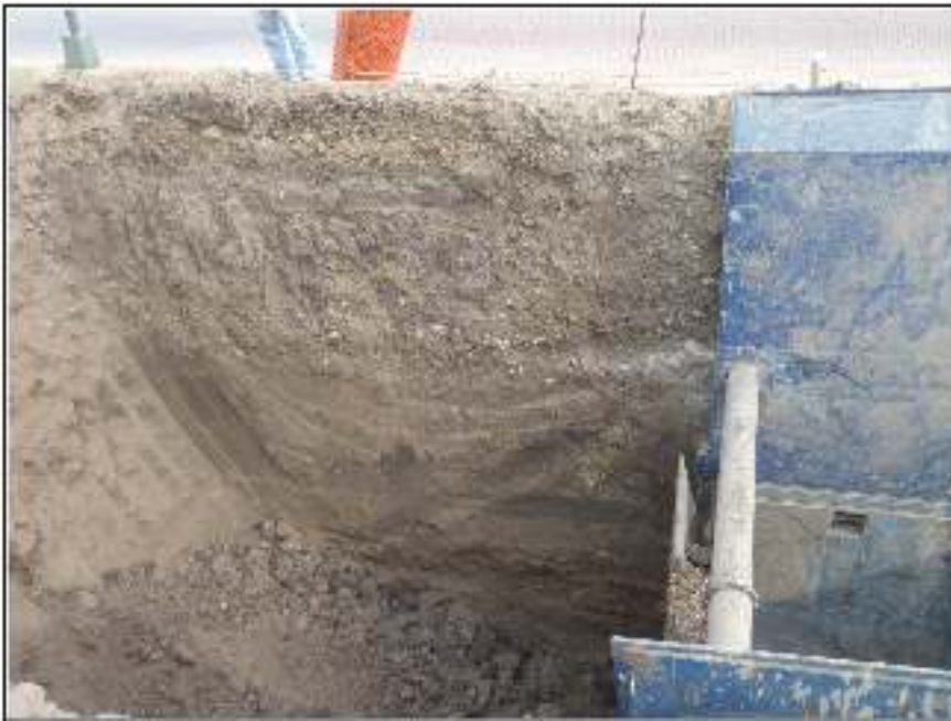
Figure 7-2. North wall profile exposed before moving the shoring unit.
