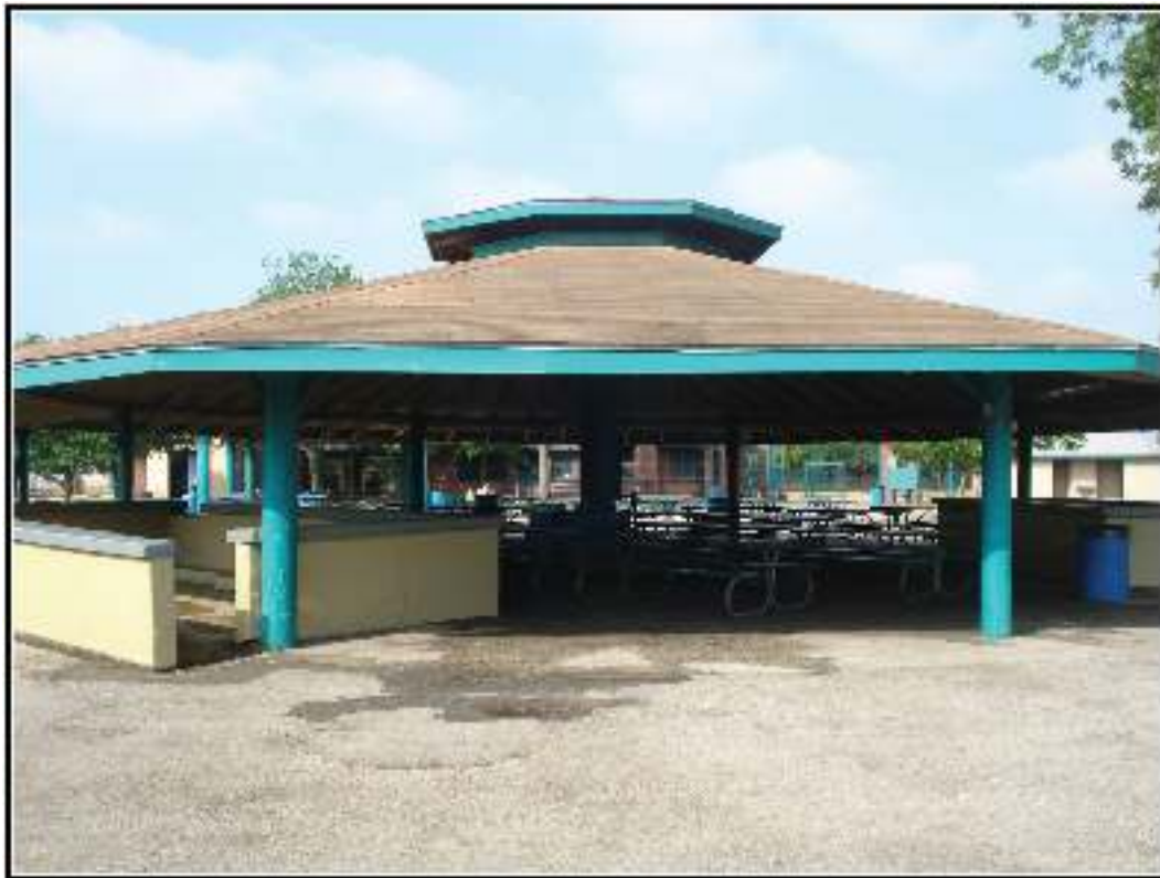
Figure 5-2. Historic pavilion structure.
