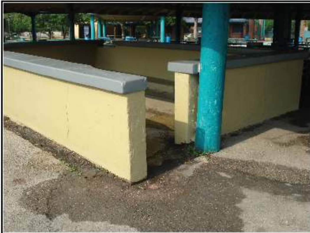
Figure 5-6. Concrete wall delineating vending area under pavilion.
