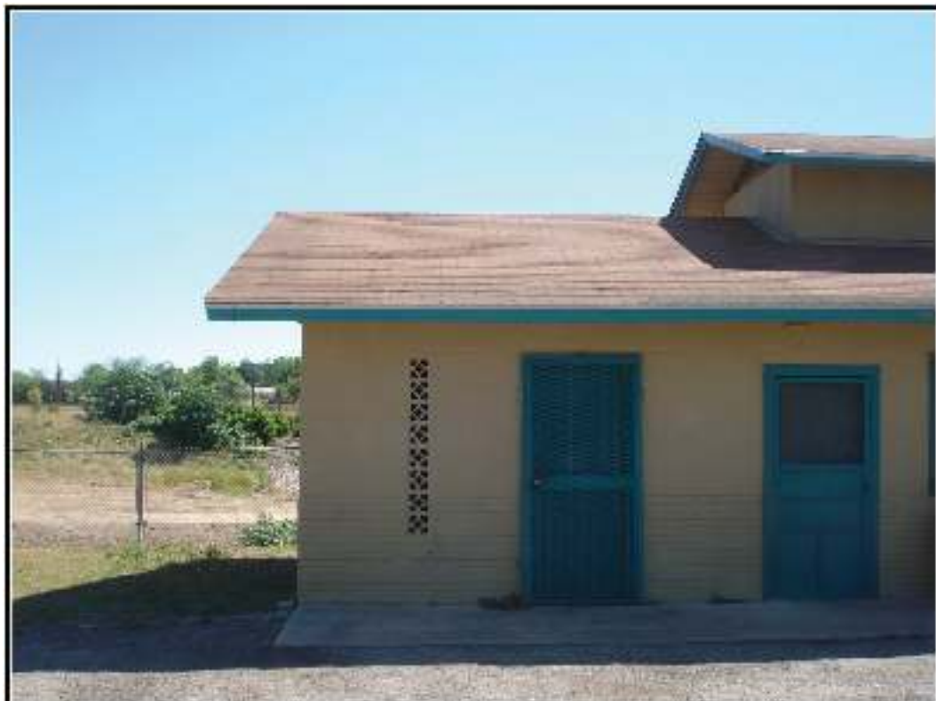
Figure 5-17. Doors and decorative detail in brick wall of rectangular brick building.
