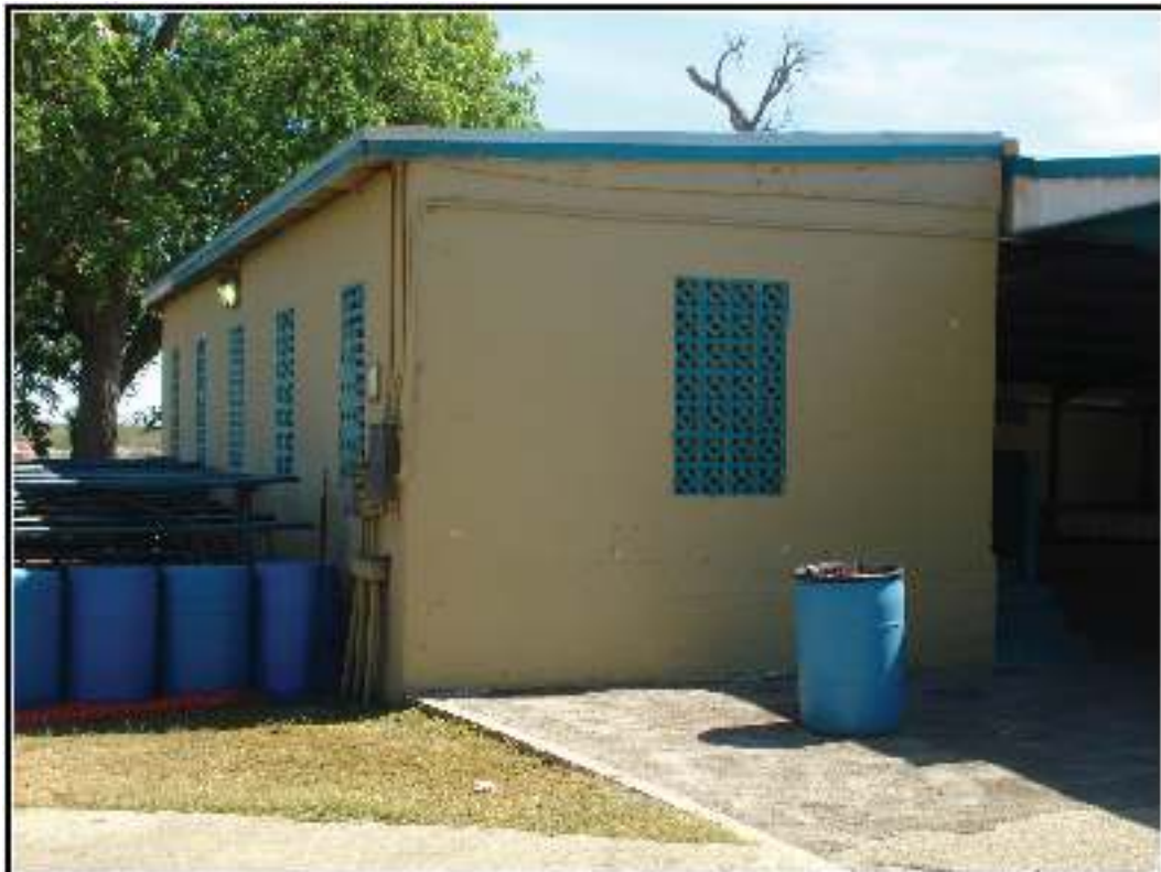
Figure 5-13. Small concrete block building attached to structure 2. Note decorative window details.
