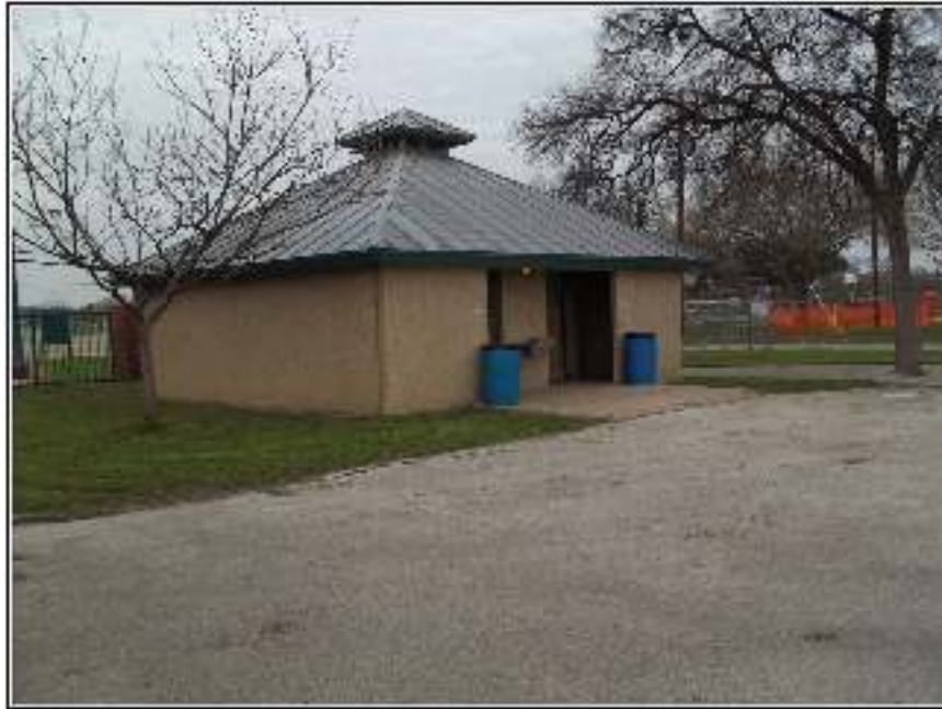
Figure 5-20. Restroom facilities within the administrative complex.
