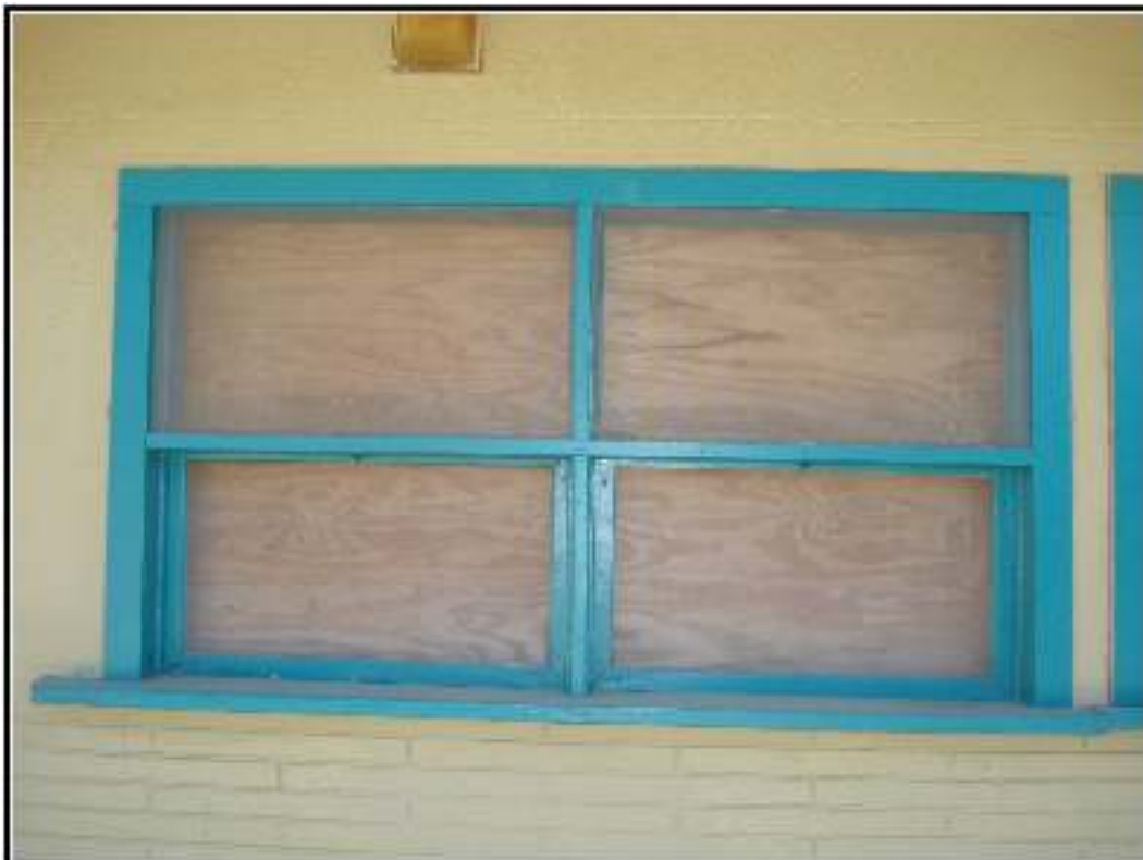
Figure 5-19. Window detail of rectangular building at eastern edge of administrative complex.
