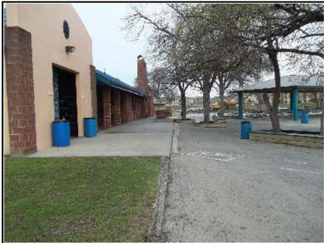
Figure 5-8. Northern end of principal administrative structure (1), looking south.
