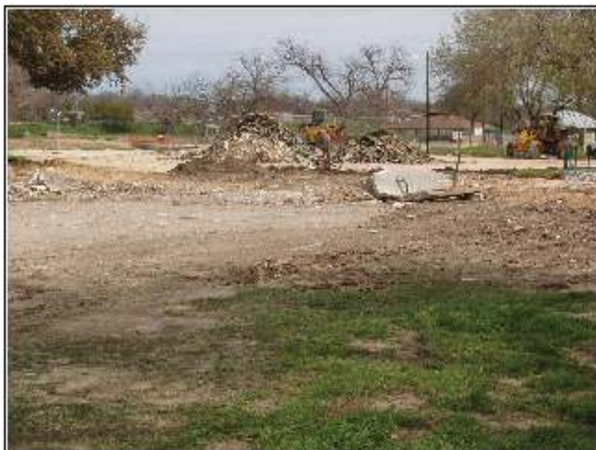
Figure 5-21. Tennis and basketball courts being demolished.
