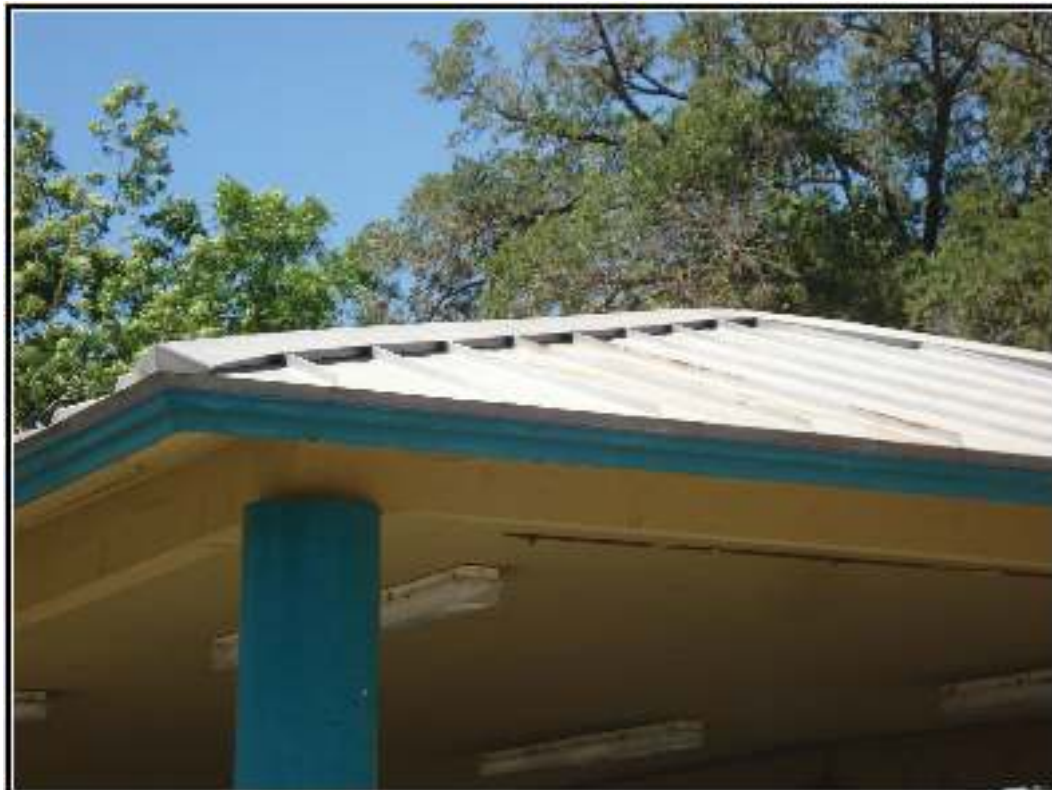
Figure 5-15. Roof detail of pavilion structure 3.
