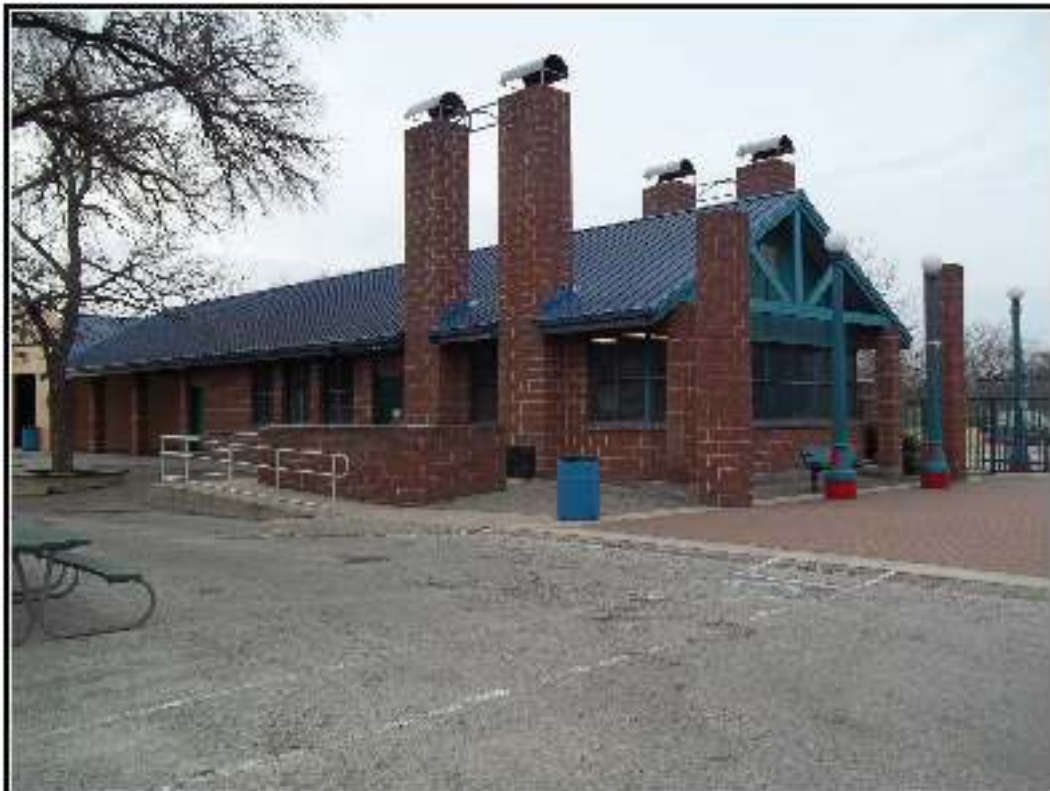
Figure 5-7. Principal administrative structure (1) that will not be demolished, looking north.
