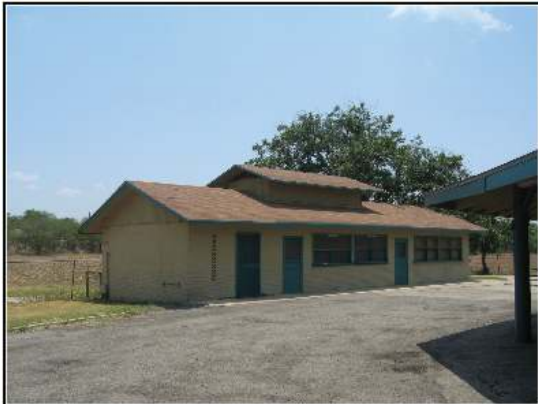
Figure 5-16. Rectangular brick building at eastern edge of complex.
