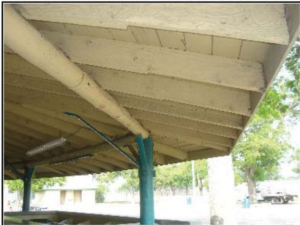
Figure 5-5. Telephone poles supporting joists and roof of pavilion.
