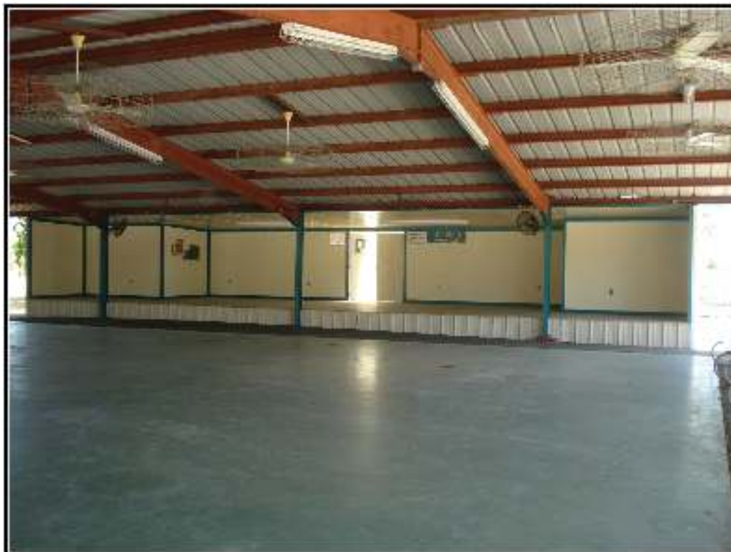
Figure 5-11. Stage-like feature at one end of structure 2, a covered pavilion.
