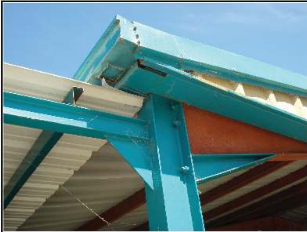
Figure 5-10. Roof detail of pavilion structure 2.
