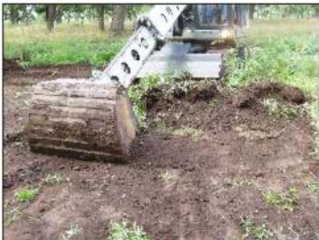
Figure 4-8. The Gradall bucket was floated in order to grade in 10-cm intervals.
