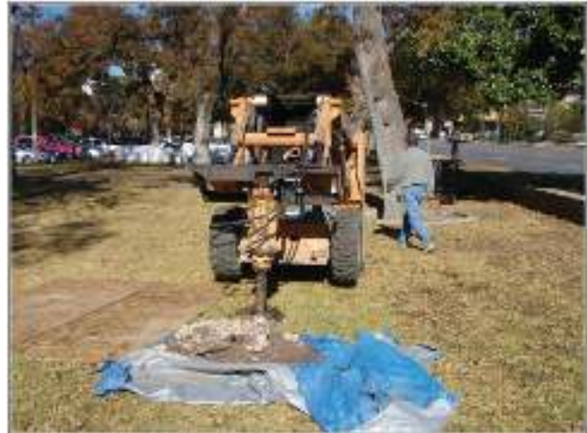
Figure 5-19. Excavation of Auger Boring 2 just north of BHT 9.
