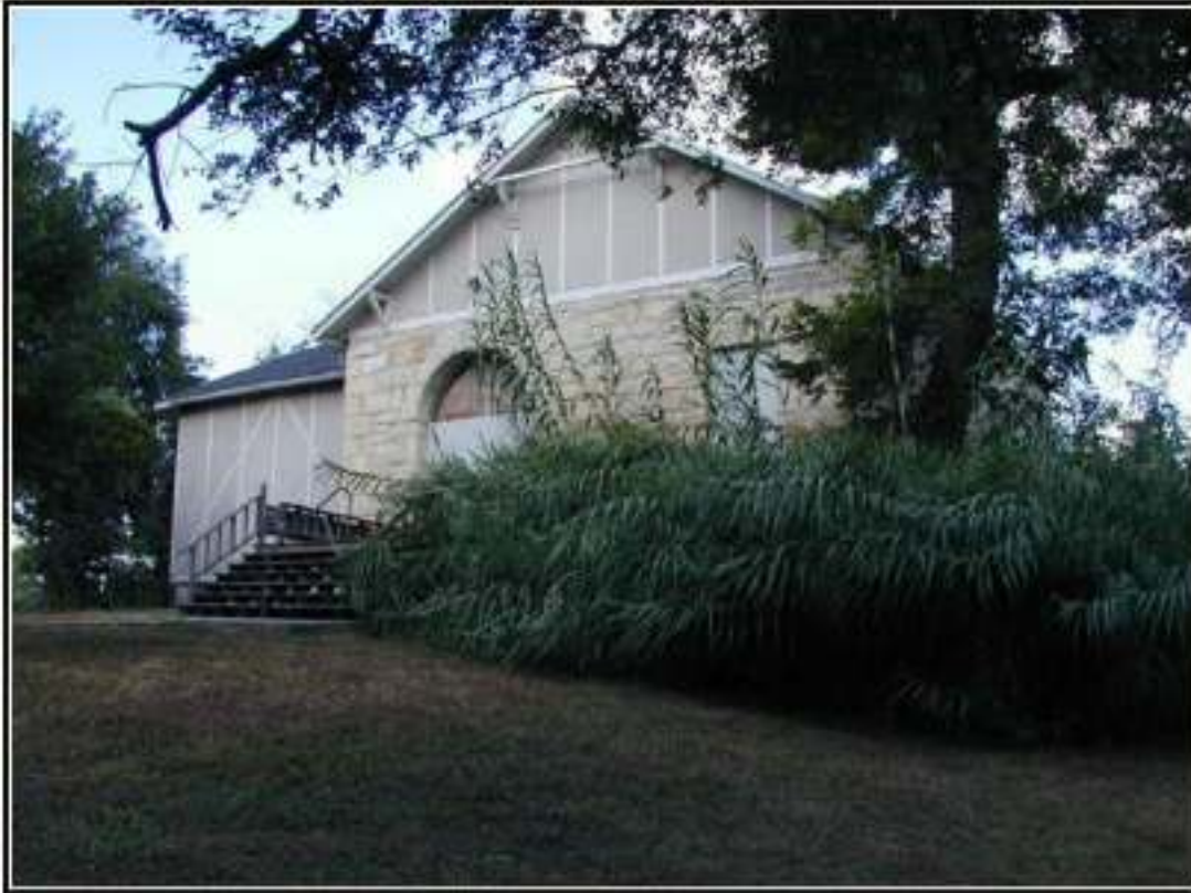
Figure 3-5. The San Antonio Water Works Pump Station No. 2.
