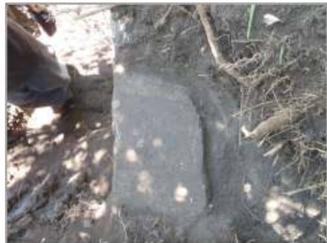
Figure 5-7. Top of the stone wall in BHT 23, facing north.
