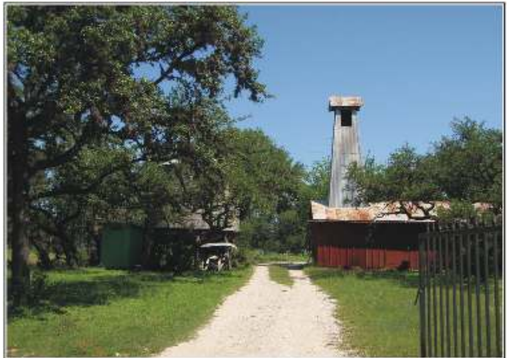
Figure A-5. The cistern and pump house on the Steubing Ranch in May 2010.
