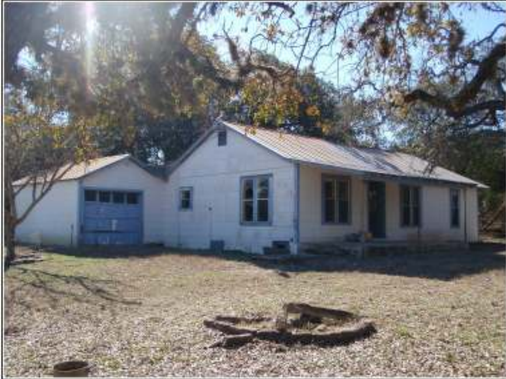
Figure 5-8. The wood-framed house within site 41KE215.
