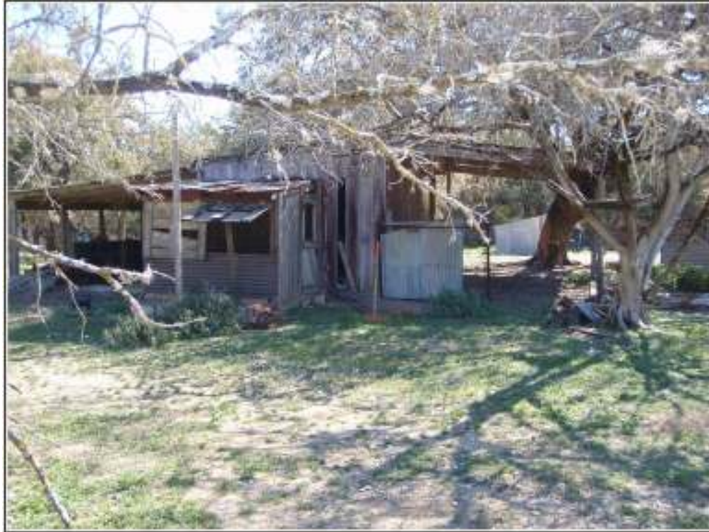
Figure 5-10. Photograph of the animal pen, chicken coop, and covered patio structure located to the northeast of the house. Facing east.
