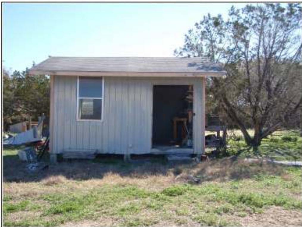
Figure 5-9. The workshop located to the northeast of the house. Facing east.
