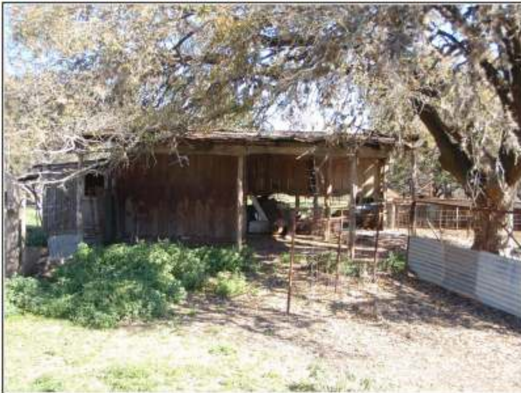
Figure 5-11. Photograph of the animal pen portion of the structure. Facing north.
