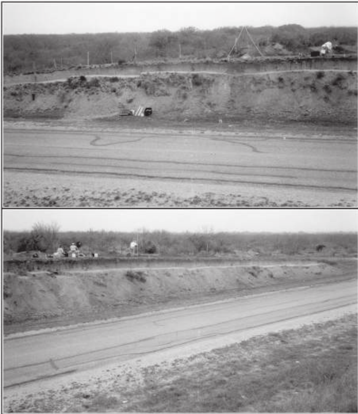
Figure 4-5. Cleaned 75 meter road cut profile. Note dark staining near top and areas of disturbance. Color images of selected sections are available in Appendix A.
