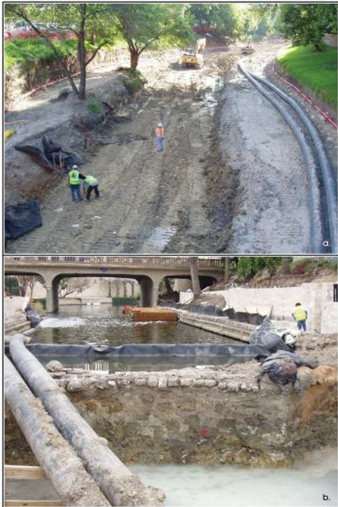
Figure 1-5. Piping river-water around the construction zone: a) river-water bypasses construction in pipes seen on the right; b) returning the water to the river at the Lexington Avenue (Hugman) Dam.
