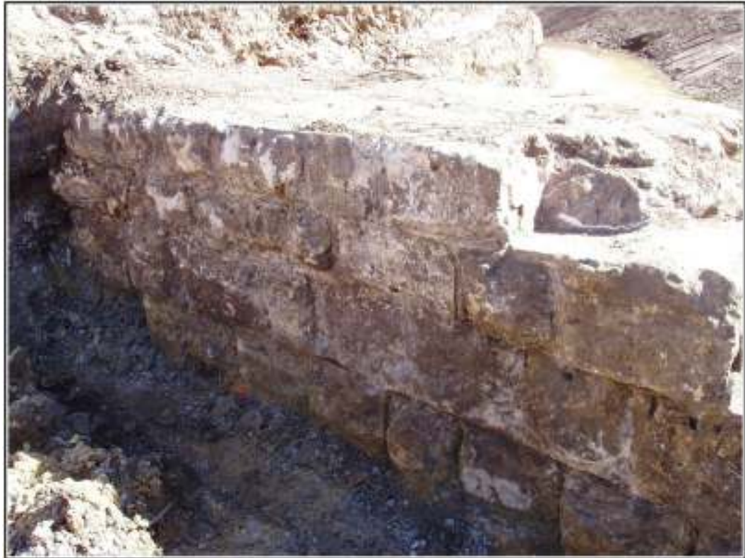
Figure 4-9. Detail of limestone blocks used to complete the Alamo Mills Dam.
