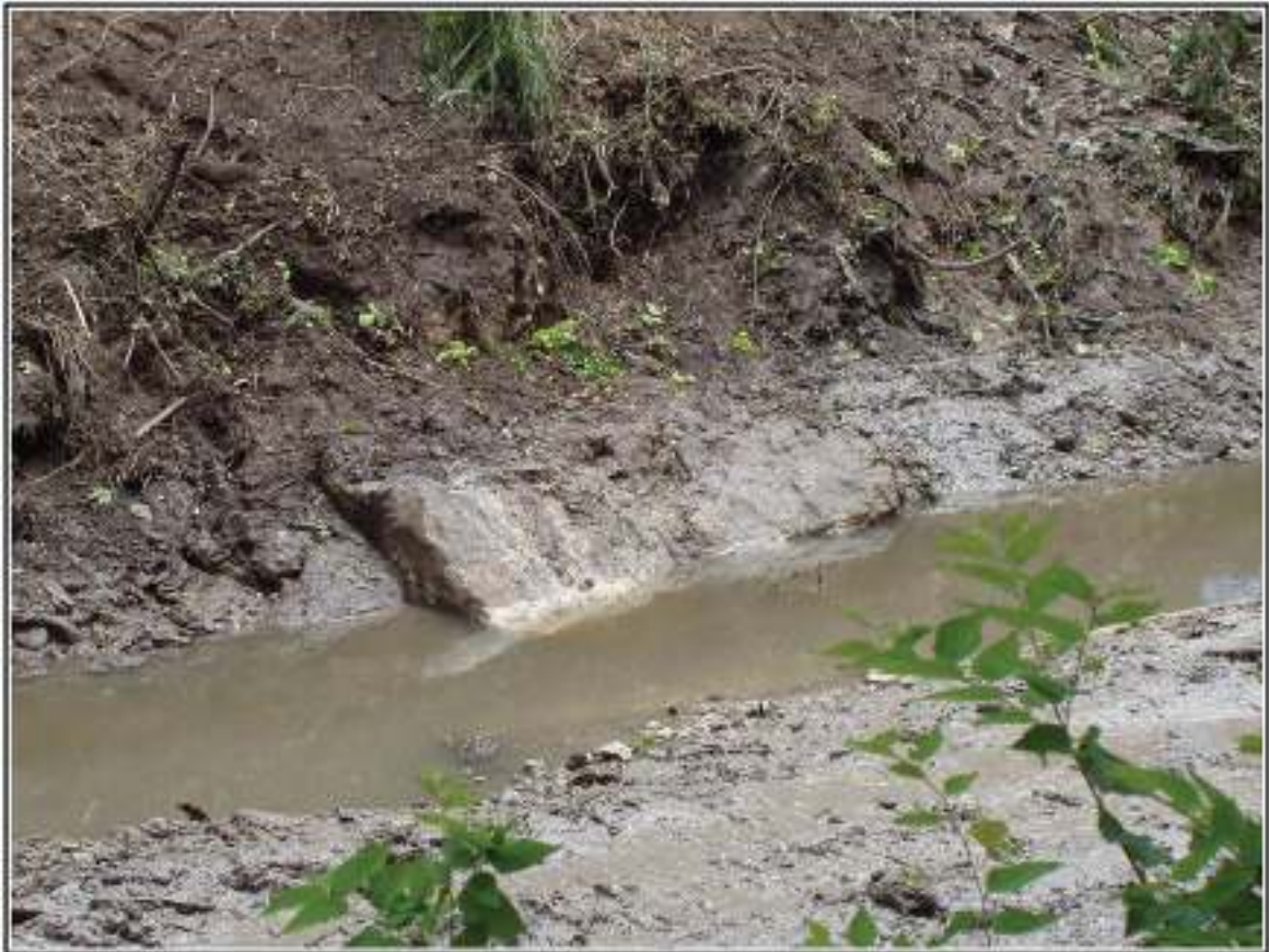
Figure 4-3. Alamo Mills Dam (41BX1817) when first encountered.
