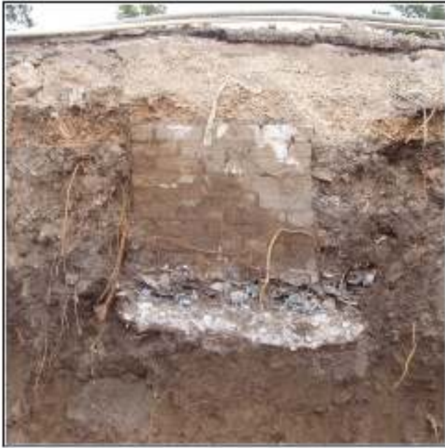
Figure 4-22. Feature 9, a brick wall with glass at the base (see Figure 4-1).
