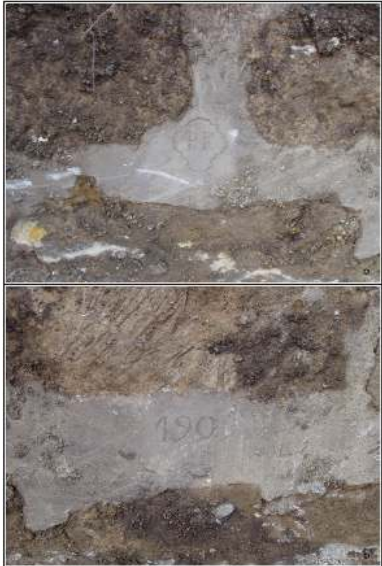
Figure 4-24. Cement in Feature 10 with notation "P.F. 1909".
