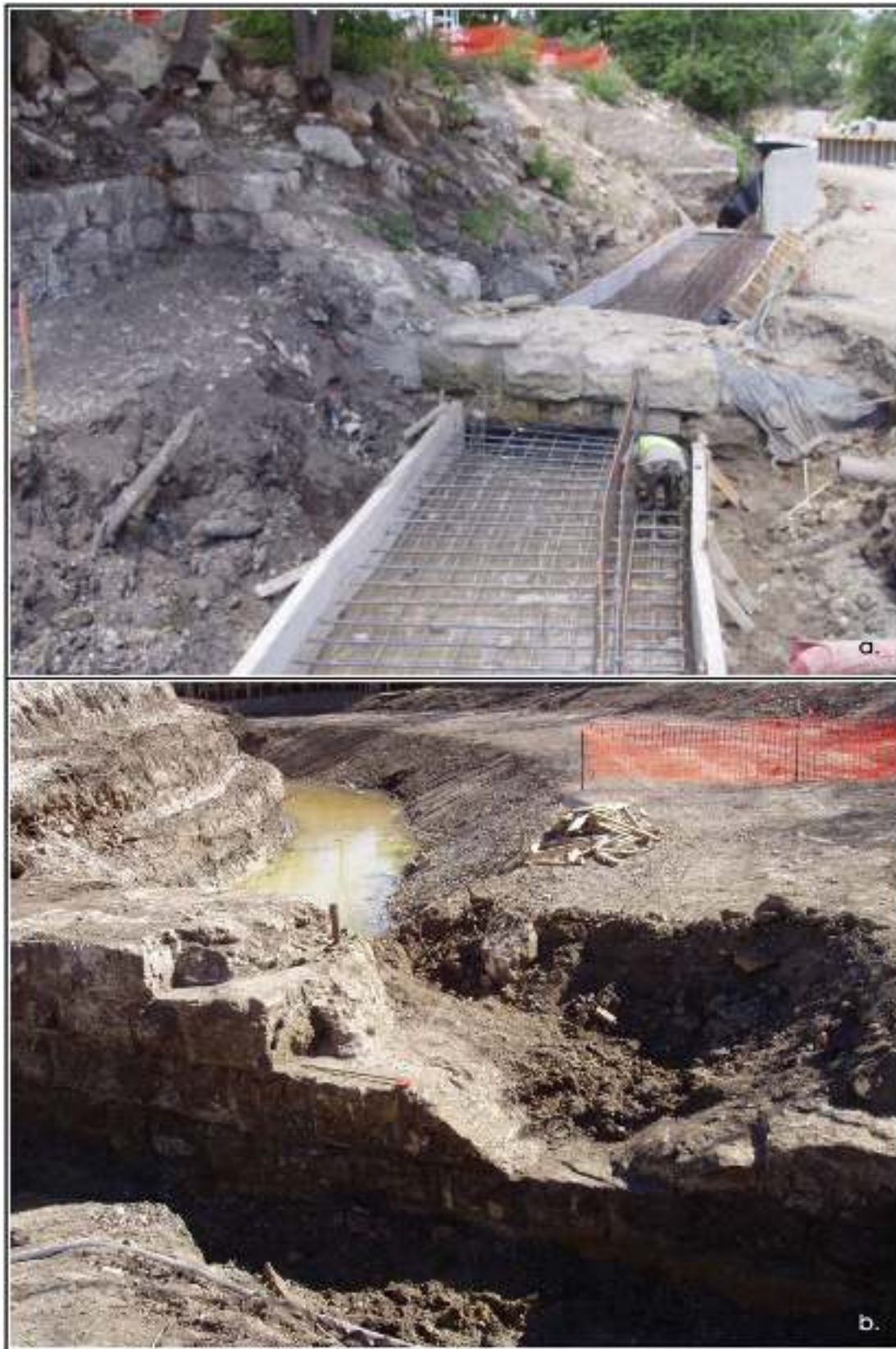
Figure 4-8. The Alamo Mills Dam after it was uncovered in 2008: a) protruding from the east bank; b) coming from the west bank.
