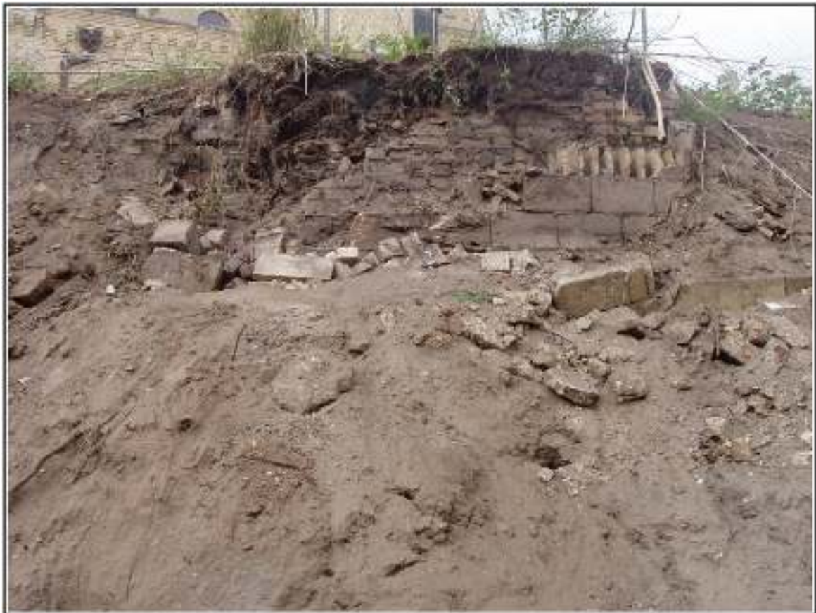
Figure 4-16. Feature 5, brick wall (see Figures 4-1 and 4-12).
