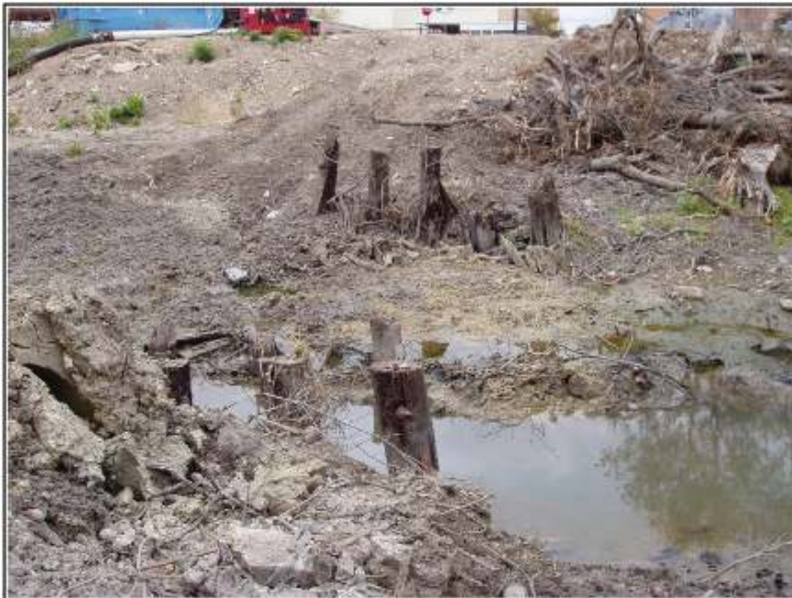
Figure 4-11. Railroad trusses located near Camden Avenue and Newell Street.
